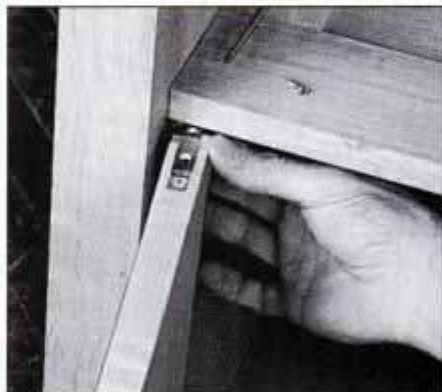
25 The doors and hinges are installed in stages. Hinges are installed in the case, and the door is slid into them.
