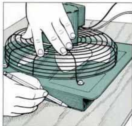
3 To mark for the fan cutout, center the fan on the plywood panel and trace around the fan's shutter housing.
