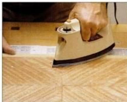
15 Use a household electric iron set at moderate heat for remelting glue in areas that may have become unstuck.
