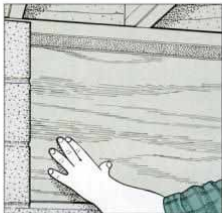
2 Cut a 3/8-in. exterior plywood panel to fill the window opening, and test fit it. This panel will support the fan.
