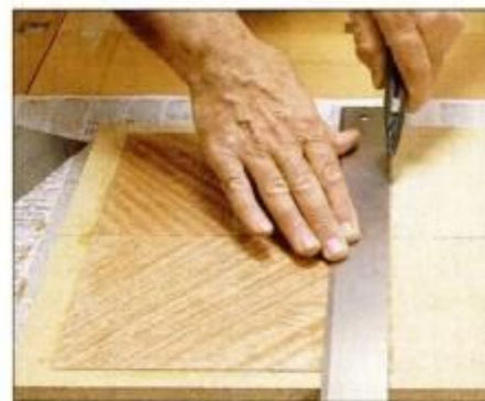
14 Use a utility knife and straightedge to true joint-line edges that may have expanded due to glue absorption.
