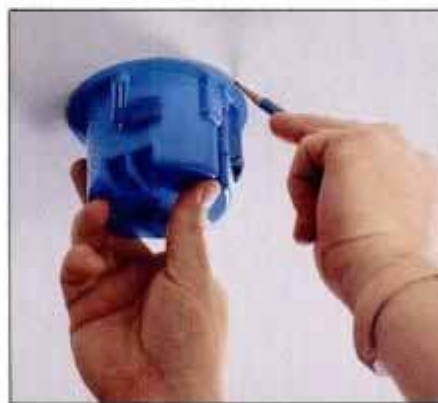
8 Hold a cut-in box to the ceiling and trace around it with a pencil. Center the box location between the ceiling joists.
