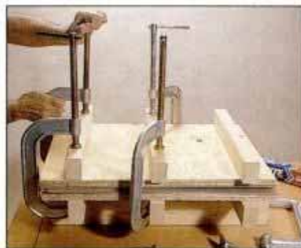
24 Sandwich panel between plywood cauls and clamp. Slightly crowned cross-bearers distribute pressure evenly.
