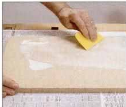
22 Apply glue to ground only. Plastic spreader makes good glue applicator. You could also use a short-nap roller or brush.
