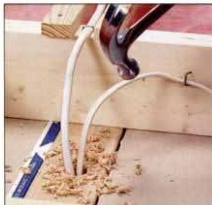
5 Staple all the cables that run along the joists. Protect cable running across joists with furring strips on either side.
