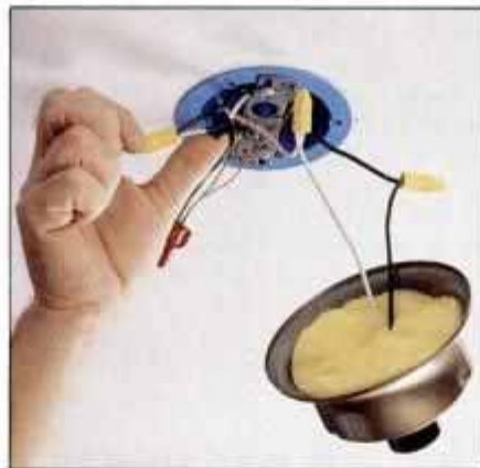
11 Join the neutral to the neutral fixture lead, hot to white switch loop, and black switch loop to black fixture lead.
