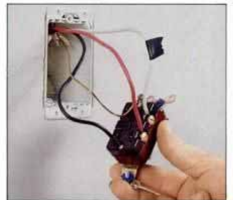
15 At second switch, the black wire goes to common terminal. Connect red and white wires to remaining terminals.
