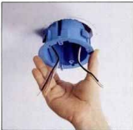
10 After removing cable sheathing and stripping ends of wires, feed wires into box. Then, mount the fixture box.
