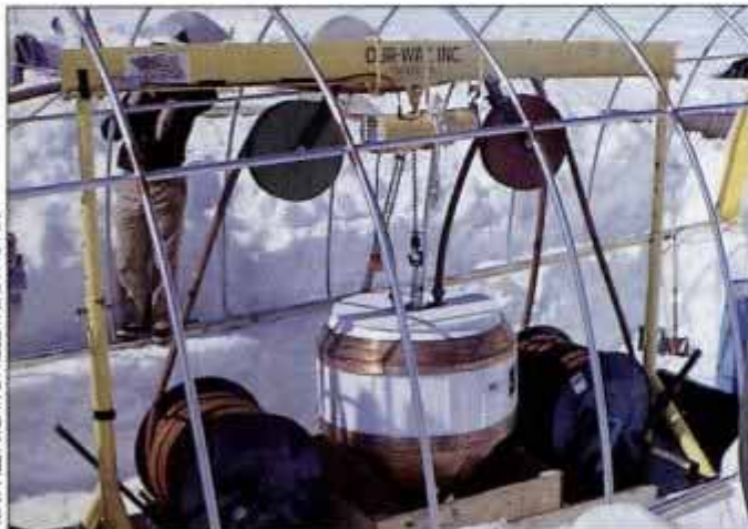
Super Gopher hangs inside partially completed work tent.
