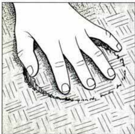
5C Cut replacement plug from hidden carpet and press plug into hole. Brush surface to blend fibers together.
