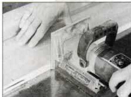
1 Place the sawn and jointed strips for the case body on the table saw. Cut the plate slots in the strips with a plate joiner.
