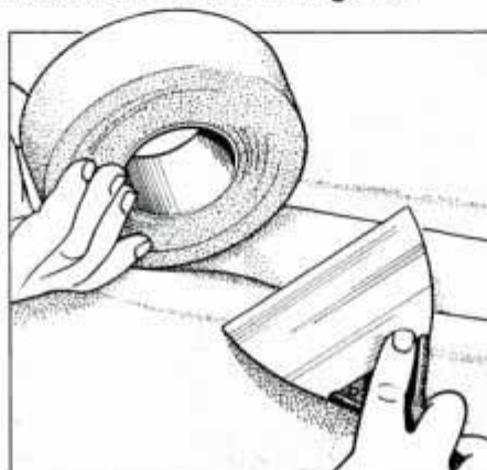
1C Imbed paper drywall tape into the compound, centering the tape over the crack. Wipe away excess and let dry.
