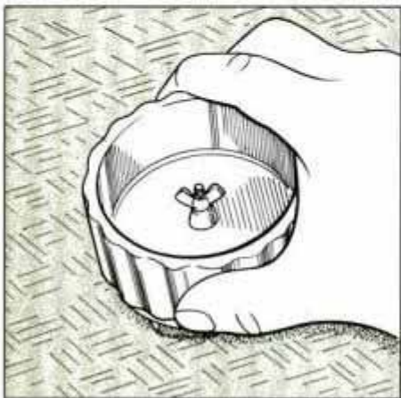
5A To remove a small damaged area of carpet, use a carpet repair cutter. Press cutter gently and turn until cut is completed.
