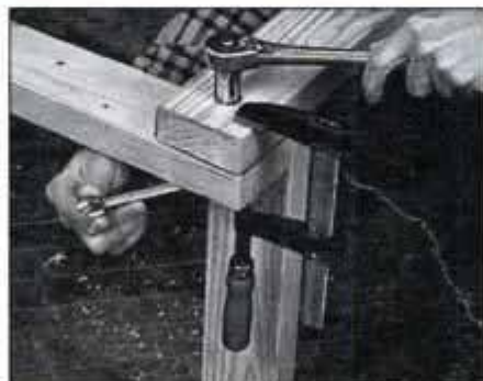
3 Use 3/8-in.-dia. × 3 1/2-in.-long hexhead bolts, washers and nuts to attach rear stringers to upright sections.
