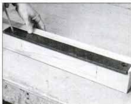
18 After laying out mortises on vise core, rout upper guide plate mortise and hold bar in place to mark bolt hole locations.
