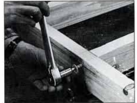
3 Temporarily clamp or nail shelf and top cross supports to frame. Then, bore pilot holes, and secure with lagscrews.
