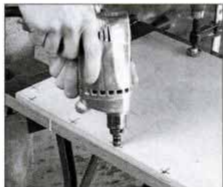
2 After laying out box screw locations so they're centered ¼ in. from edge, bore and countersink screw pilot holes.
