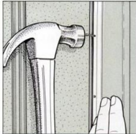
5 For doors that aren't warped, but fit the jamb poorly, use vinyl tube weatherstripping with extruded aluminum flange.
