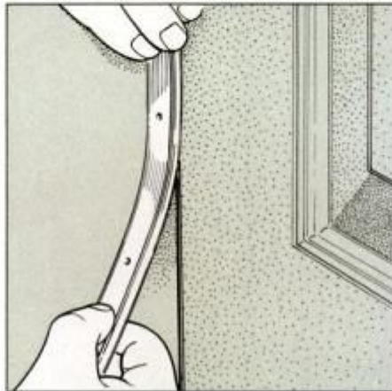
4 To seal a warped door, nail vinyl tube weatherstripping to the doorstop. Bend the tubing to follow the door's curve.
