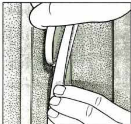
2 Peel off backing paper from under vinyl V-strip, and smooth it in place. Do the top jamb first, then do the side jambs.
