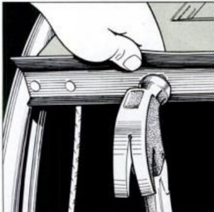
11 Remove worn-out garage door weatherstripping. Prime and paint door bottom, and nail on the new gasket.
