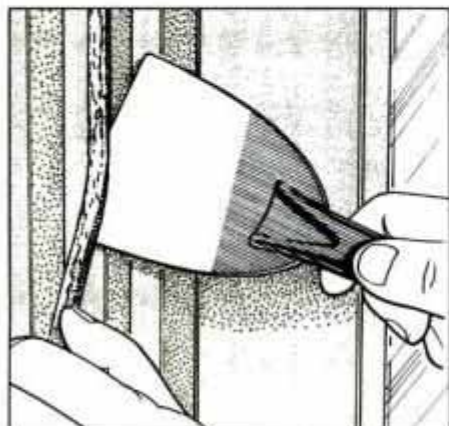
1 Pry loose old weatherstripping with a wide putty knife. Wash the doorjamb, and scrape off loose paint. Prime bare spots.
