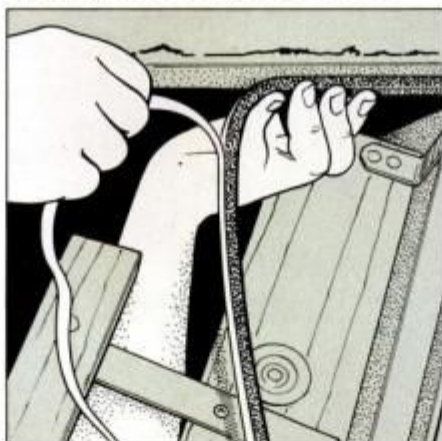
9 Apply \frac{1}{4} -in.-thick adhesive-backed foam rubber to the jamb of disappearing attic stairs to stop air leaks.
