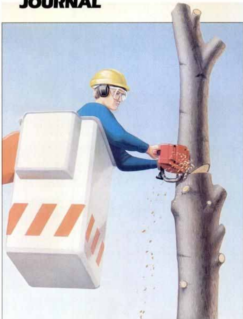
Felling a tree in a residential area requires experience and the right equipment. The first step is to remove the branches from the bottom up. Then, the tree is cut down in sections.
