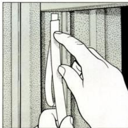
15 Pinch legs of the V-strip flat, and poke end with folded backing paper into the small space between window and jamb.
