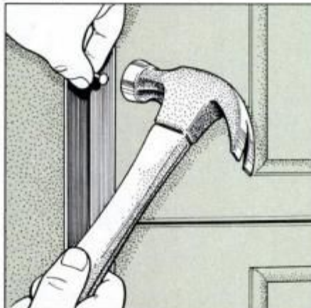
12 Nail flexible vinyl weatherstripping to garage doorstop to seal the opening. Press strip firmly against door as you nail.
