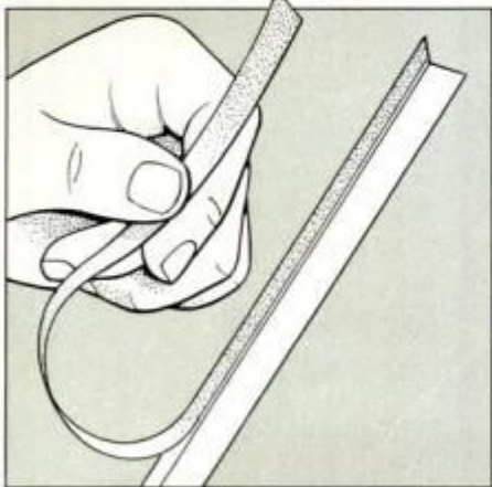
14 Begin sealing inner sash by slicing backing paper about a foot down from top of V-strip. Fold paper back on itself.
