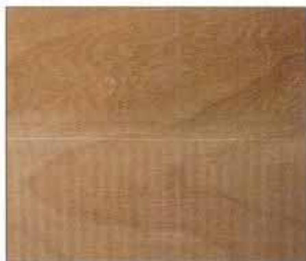
3 Although not obvious during construction, milling marks will show up after finishing (below). Top half is scraped flat.
