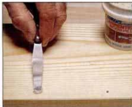
7 Cover set nailheads with wood filler. Remove excess while leaving just enough filler to sand flush with wood surface.
