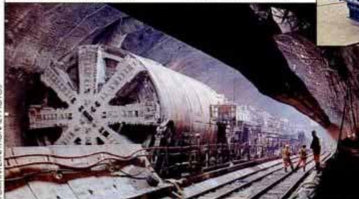
Channel tunnel's boring machines (top and bottom), more than 600 ft. long, are burying themselves. Monster compressor (right) is heart of cooling system. Engineers expect to have the job finished by mid-1993.
