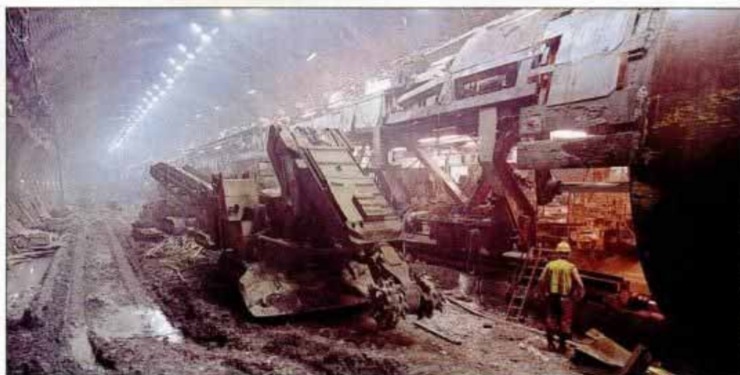
Channel tunnel's boring machines (top and bottom), more than 600 ft. long, are burying themselves. Monster compressor (right) is heart of cooling system. Engineers expect to have the job finished by mid-1993.
