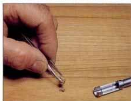
6 Make an almost invisible patch with a plug cut from a scrap of the same wood. Bore out blemish, align plug, and glue.
