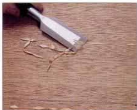
1 Remove excess glue by carefully peeling it off the surface with a sharp chisel after the glue has partially set.
