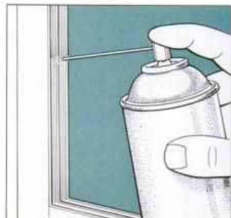
7D Lubricate the frames, latches and sash channels with a spray lubricant. Then, reinstall the sashes, and check operation.
