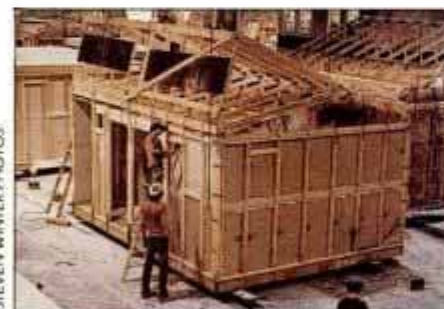
Modular homes are built almost entirely in the factory and then trucked in modules to the building site where they are erected.
