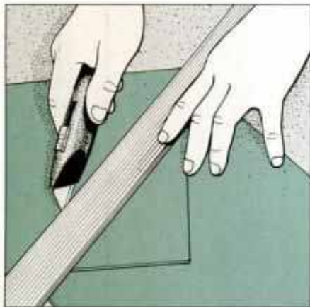
4 Where NobleSeal strips adjoin, cut a butt joint. Overlap the strips, and cut the joint with a razor knife and straightedge.
