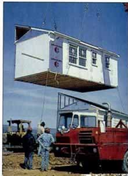
Modular homes are built almost entirely in the factory and then trucked in modules to the building site where they are erected.
