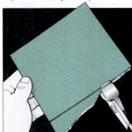
13 For a cut near the tile's edge, score first with the tile cutter, then use tile nippers to nibble up to the line.
