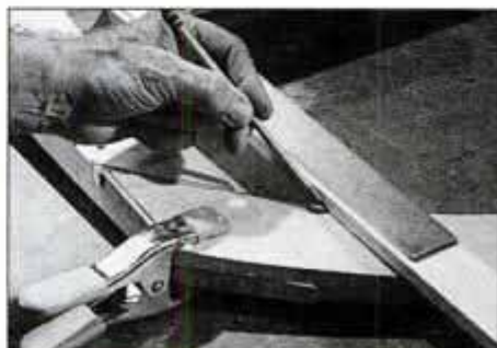
19 Ensure perpendicular alignment of slats in bottom rail with a framing square. Mark slat positions on arched rail.
