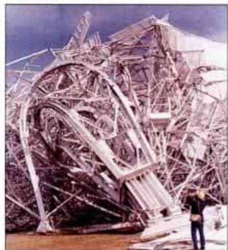
Spontaneous collapse of the 30-year-old observatory gave rise to a new design.
