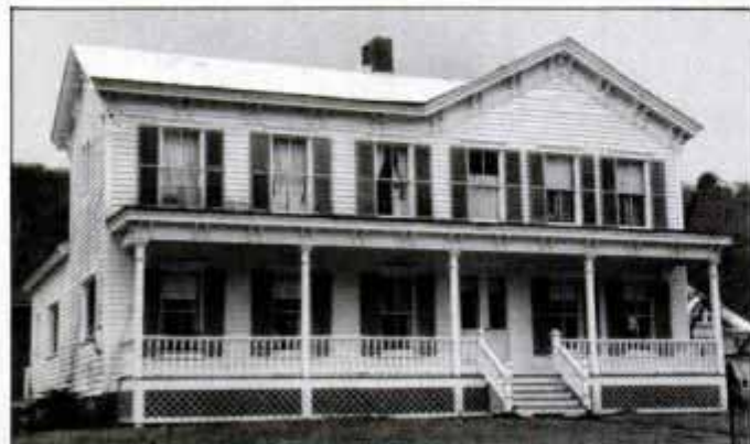
The original front porch, with tapered and chamfered columns, rich molding details and stately proportions, forms the inspiration for our reproduction back porch project.
