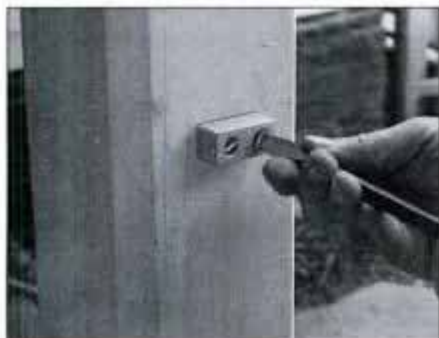
34 Screw rail-support blocks where upper rail meets posts or house walls. Slide rail assembly in place and toenail.
