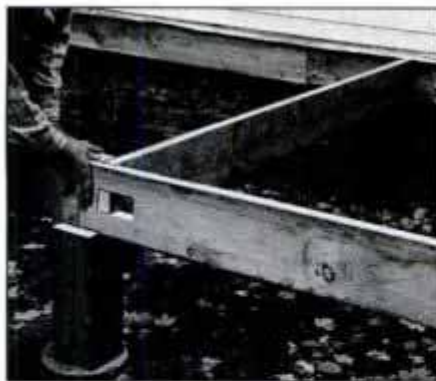
7 Test fit inner main beam with single crossbeams and posts. Then, add outer main beam with nails and construction adhesive.
