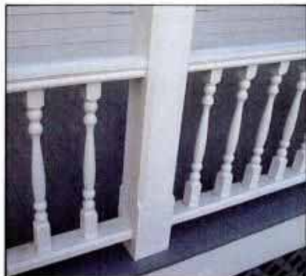
The rails are made from ordinary lumber that's shaped to the original design. Balusters are standard pressure-treated type.
