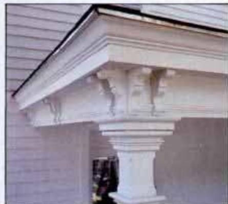
Our reproduction moldings capture the shape and depth of the originals, but are assembled from profiles made with a router.
