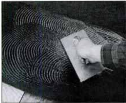
25 Apply appropriate roofing adhesive with a notched trowel to secure each course of roll roofing to the last.
