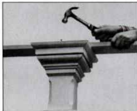
20 Begin roof construction by nailing beam bottom trim to post tops. Butt trim at posts and miter at corner post.
