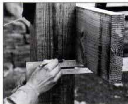
6 Temporarily nail or clamp single crossbeams at correct height to 6 x 6 posts. Mark the post notch line with square.
