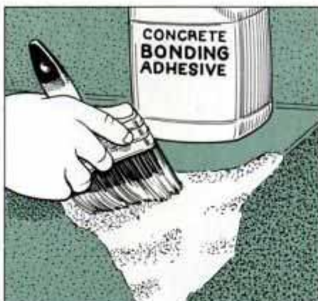
1B Use a paintbrush to apply concrete bonding adhesive to the damaged area. A synthetic bristle brush works best here.
