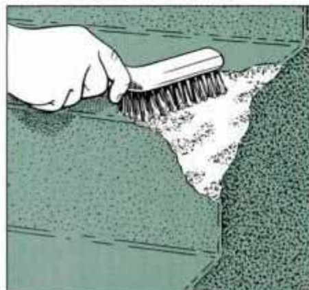
1A Clean away debris on damaged concrete with a wire brush. Concrete patch will bond poorly unless corner is prepared.
