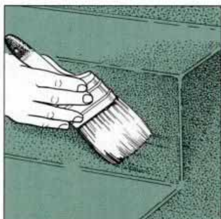
1E Remove form and smooth over patch with a wet paintbrush. Avoid patch until it is fully hardened in a few days.
