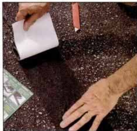
1 Unroll Driveway Medic along the length of the crack, cut it to length with a razor knife, then peel off backing paper.
