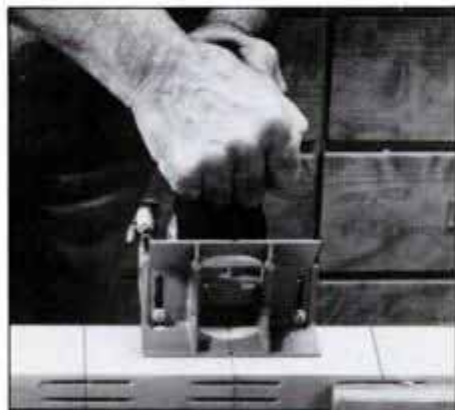
3 Secure workpiece in a vise to quickly and safely cut the slots. Align fence by eye, and plunge cutter into the workpiece.
