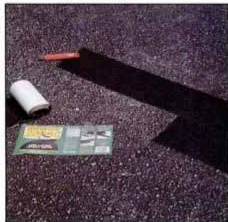
2 Press the patch over the crack. Use more than one piece for large cracked areas. Seal over the patch if you wish.
