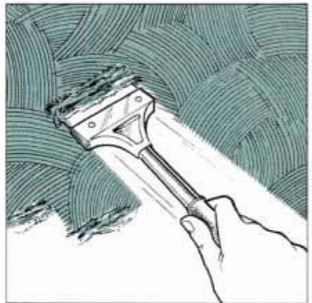
A simple wallpaper scraper with a razor blade does a great job removing old adhesive. Always push the tool away from you.
