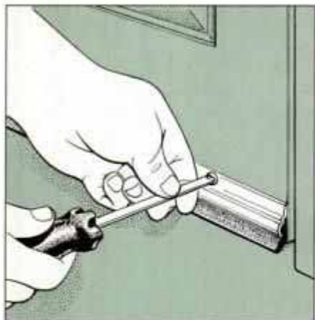
Inspect all door sweeps for fit. If they are loose, tighten them. But if worn, replace them with new layered vinyl versions.
