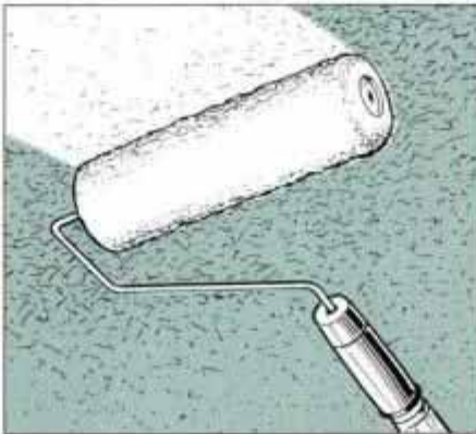
Textured surfaces, like ceilings, generally absorb paint unevenly. To prevent this, roll on an alkyd primer before painting.
