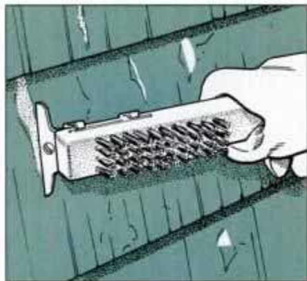
13 Once windows are repaired, return to sliding and hand scrape any loose paint that was too stubborn for power washer.
