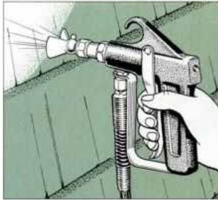
23 Begin spraying building at top and moving across and down. Keep spray head perpendicular to surface at all times.
