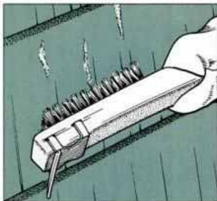
14 Once paint is scraped off, brush exposed areas with wire brush. Brushing loosens paint that scraper blade missed.
