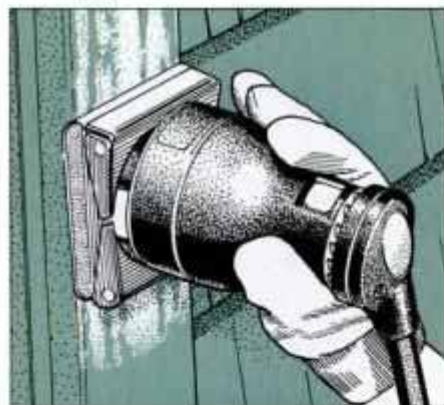
16 On surfaces where lots of paint has been removed and exposed wood is rough, sand surface smooth with palm sander.
