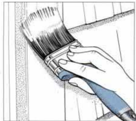
27 Once sash is painted, coat jamb and window trim. After all windows, doors and trim are painted, spray rest of siding.
