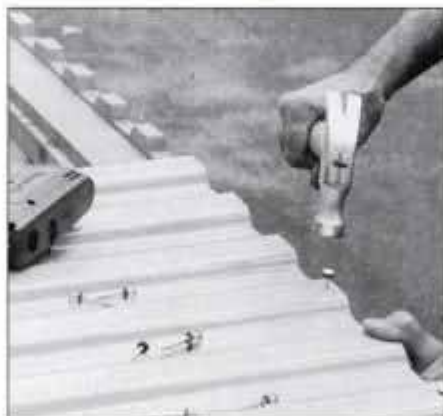
20 Prebore clearance holes in panel ridges and molding. Attach panels with aluminum nails that have rubber washers.
