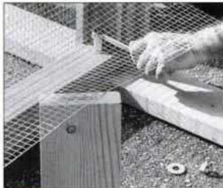
11 Don't nail mesh at the bottom of the two center frames so you have access to nut. Tighten the nut until bolt digs in.
