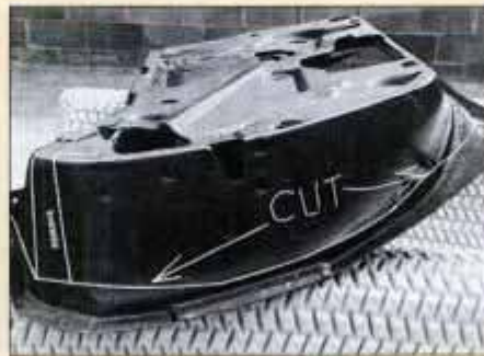
Metal door assembly is modified by cutting components with a die grinder and then re-assembling. Welding is necessary.
