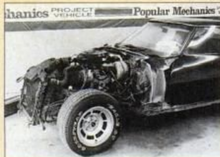
Front clip is removed as a unit after cutting cowl area and separating fenders from cowl by prying apart factory epoxy bond.
