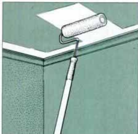
12 Use a 4-ft.-long extension handle when painting ceiling and walls. The extension screws into the roller handle.
