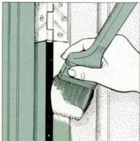
16 Paint door's side, top and bottom edges. Cut in cleanly around hinges, avoiding drips. Next, paint the door jamb.
