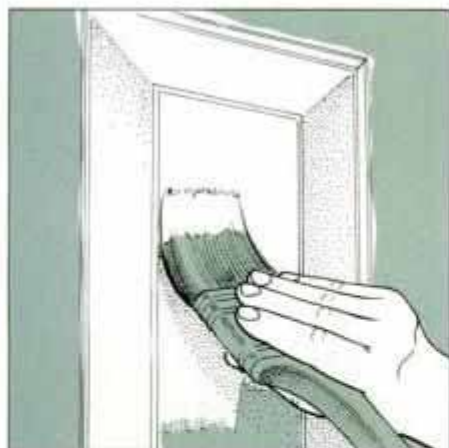
13 Next, work from the top down and paint the panel's face. Work the paint into outlined area to prevent lap marks.
