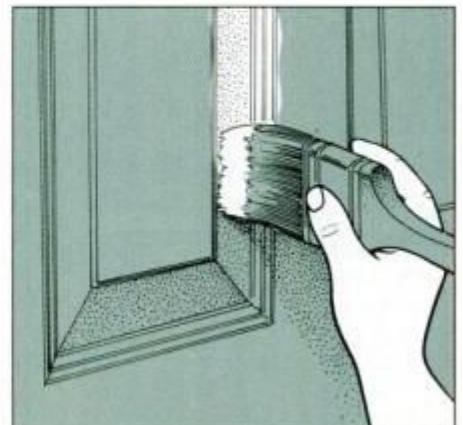
12 Start painting a paneled door by outlining the molding around each panel. Use a 2½-in.-wide, square-tip brush.
