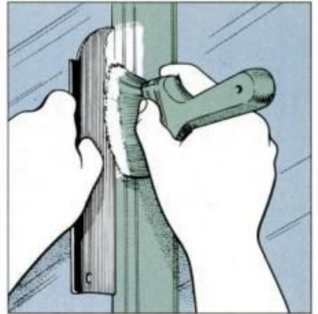
6 You can also keep glass free of paint with a trim guard. On bare wood windows, allow some paint to seal against glass.
