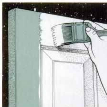
15 Paint the top and bottom rails and then the outside stiles. Paint the long surfaces with a continuous stroke.
