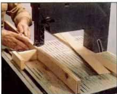
9 Resaw the 3/8-in.-thick deck slats from 3/4-in.-thick stock. Smooth away the saw marks by planing or sanding.
