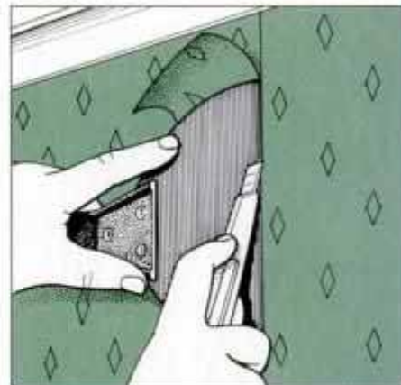
18 To make a double-cut joint, align the pattern with the strips overlapping. Press hard enough to cut both strips.
