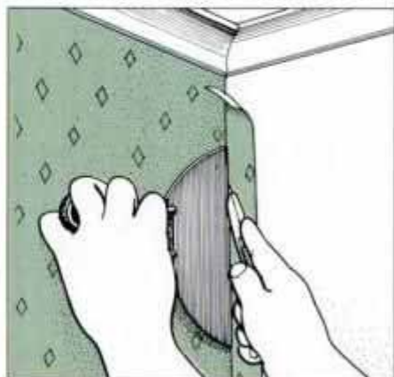
15 Trim paper flush working with broad knife and razor. This leaves a small bit of paper overlapping in the corner.
