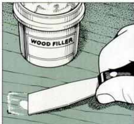
5 Firmly pack wood filler into gouges using a putty knife. Strike off the excess.
