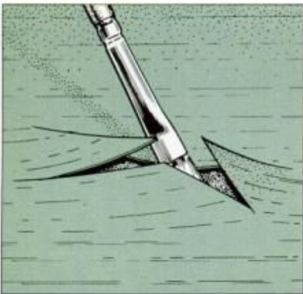
19 Make X-shaped slit on a large blister. Peel back the flaps and brush on cement.
