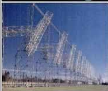
New radar (above) bounces off the ionosphere to surface. Four sites (far left) will cover North America. Each of three Maine antennas (left) is 3600 ft. long.
