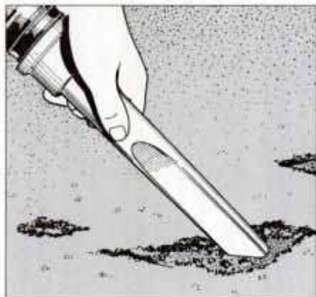
5 Loose debris can be removed from narrow holes and wide cracks using a crevice nozzle and a wet/dry shop vac.
