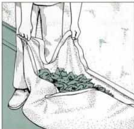
16 To complete the job, fold up debris in disposable dropcloth and throw it out. Let the walls dry before painting them.
