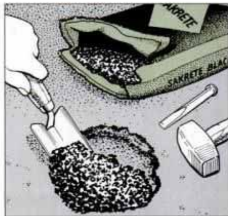
12 Remove loose pavement around large potholes by chopping it out with a cold chisel and a hammer. Trowel in cold patch.
