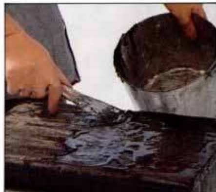
2 After about 15 minutes, scrape off old finish with wide-blade putty knife. If paint remains, repeat stripping process.
