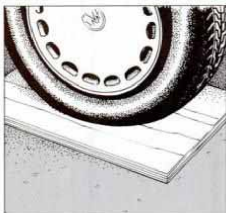
13 Cold patch must be thoroughly packed down. One method is to place plywood on patch and drive a car onto the plywood.
