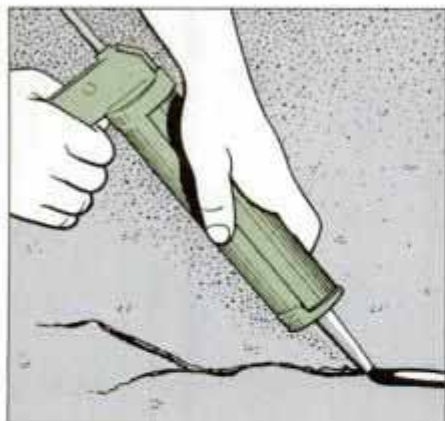
10 Driveway crack filler is used on cracks up to ¼ in. wide. Fill deep cracks with sand before applying filler.
