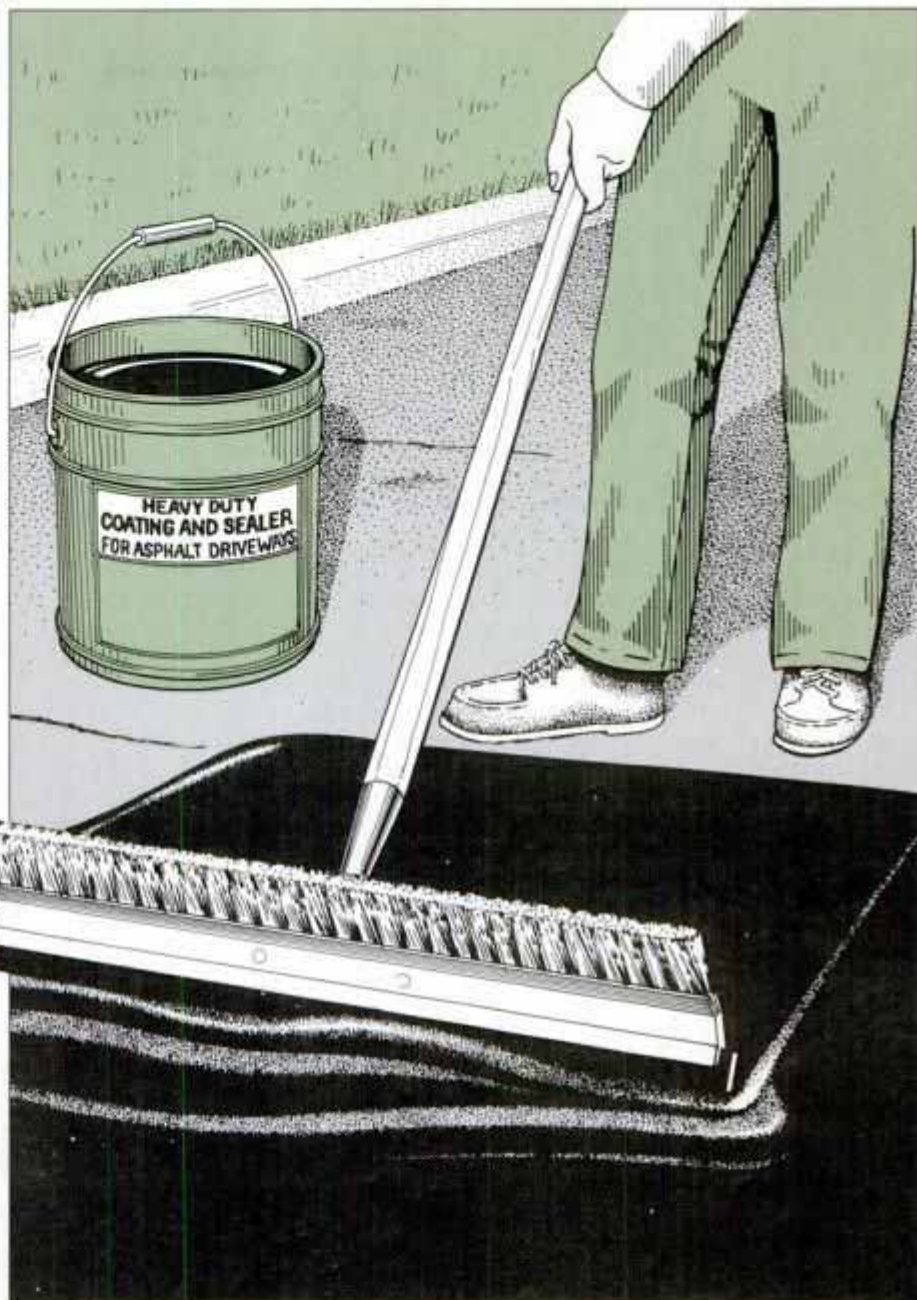
Sealing a driveway extends its life and improves its appearance. It's important to prepare it for sealing. Clean it, patch its potholes and fill its cracks, then apply sealer.
