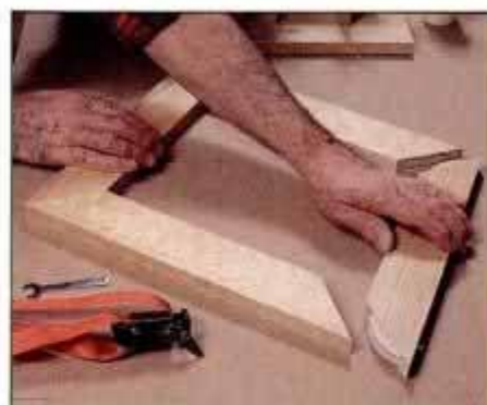
17 Here, two plates are installed at each corner of mitered frame for extra strength. Band clamp holds pieces until glue sets.
