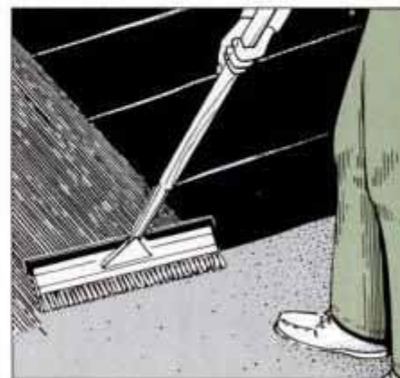
15 After sealer is evenly spread, brush at right angle to direction taken with squeegee. Work the sealer into the surface.
