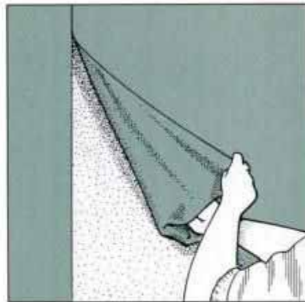
14 Pry up one corner of the strippable wallpaper using a putty knife or scraper. Slowly peel the paper off the wall.
