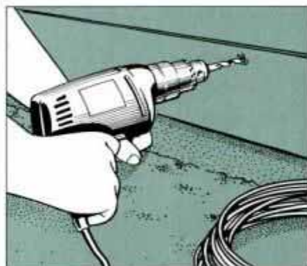
2 To bring cable from an indoor control box, bore a hole through rim joist or wall and feed the cable through the hole.
