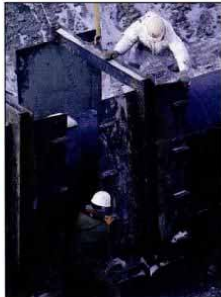
Ultrasonic probe (top left) homes in on anomalies. Then, after pipe is sandblasted, coated and taped, steel collars are lifted onto pipe (lower left), and welded (top right). In some areas, slurry is poured into forms (lower right) to guard against sharp rocks.
