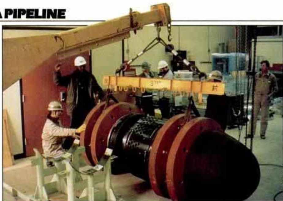
Ultrasonic pig is prepared for launch at one of the pipeline's pumping stations.
