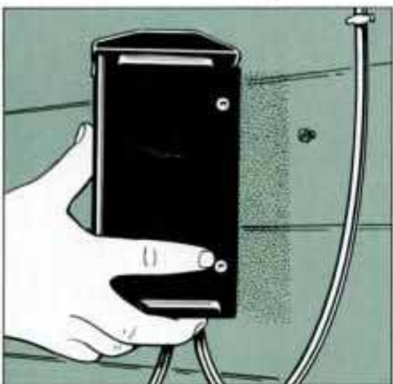
5 To mount control box, drive screw into wall (and stud behind) leaving 1/8 in. of shank exposed. Hang box on screwhead.
