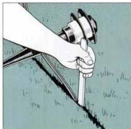
18 Force cable into spade opening with a paint stick or thin piece of scrap wood. Work gently to avoid damaging wire.
