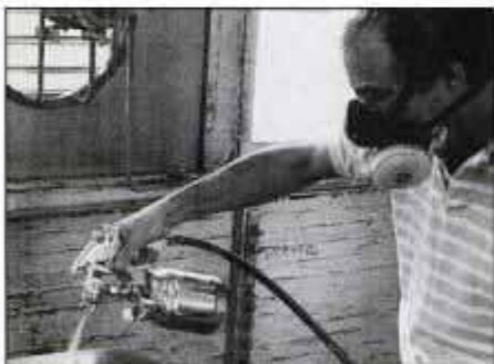
26 Primer and top coat can be brushed or sprayed. Wear respirator with cartridge rated for a naphtha-thinned finish.
