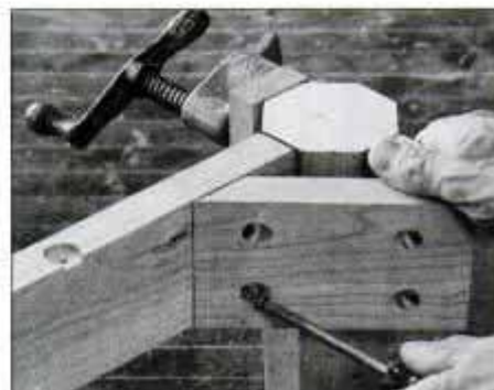
13 Glue and clamp together subassemblies with short aprons. Cut corner braces to span long and short aprons, and install.
