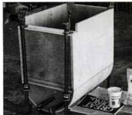
12 Glue and nail the blocking inside curved pedestal. Glue and clamp the half round to pedestal using gap-filling epoxy.
