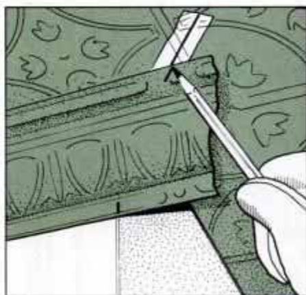
18 Hold length of cornice molding in place so that it extends past the line on the ceiling. Then, mark where the molding meets the line and the outside corner.
