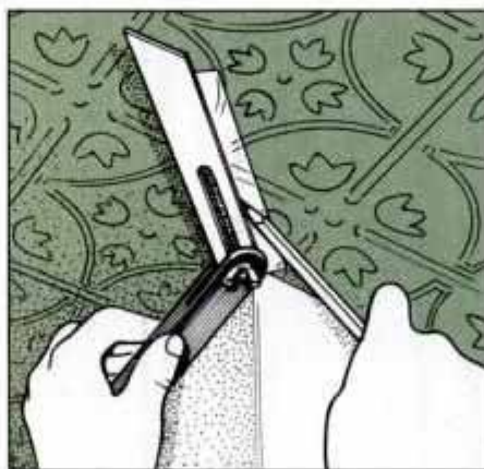
17 Bisect the angle of the outside corner and mark it on the ceiling with a pencil and sliding bevel square. A strip of masking tape shows the pencil line clearly.
