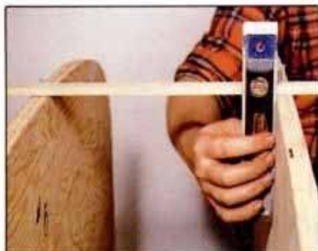
4 Tack a strip across all molds at the centerline. Adjust each mold for plumb with level. Then check molds for fairness.
