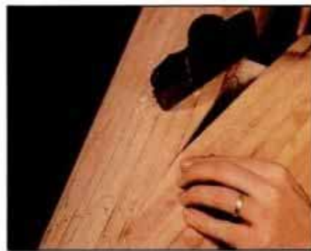
15 The remaining pieces are mitered at one end, pressed in place and marked for the miter at the other end. Cut and install.
