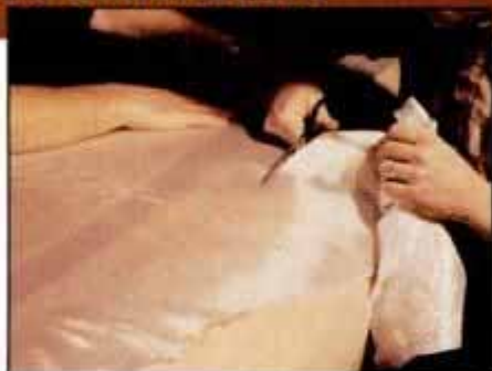
21 Begin fiberglassing by laying 38-in.-wide cloth over the hull. Cut to a football shape that matches the bottom.
