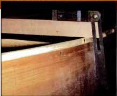
27 Lay a straightedge across center of hull and use bevel gauge to determine gunwale bevel. Then bevel outwales and inwales.
