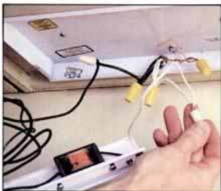
5 Locate leads in wireway. Then attach black lead to black pigtail and white lead to white pigtail using Wire-Nuts.
