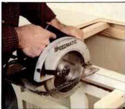
11 If countertop is too large to remove in one piece, support it on scrap blocks, then cut into pieces with carbide blade.
