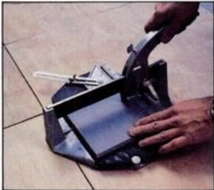
7 Cut tiles to size on tile cutter. Just score surface with arm and snap off. Tool works best when cutline is near center of tile.
