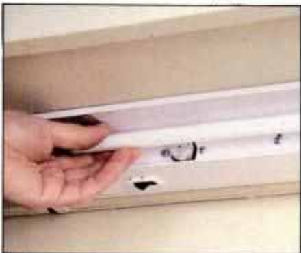
7 Push fluorescent tube into fixture brackets. Then replace plastic light diffuser. Turn on power and check for proper operation.
