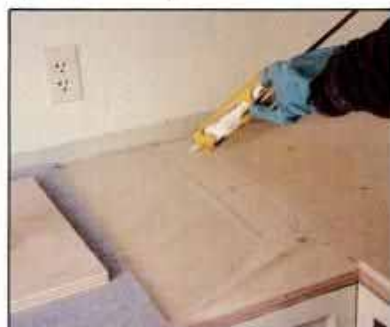
8 Join counters to substrate with dabs of silicone adhesive. Place wax paper under seams to keep seam area from bonding.
