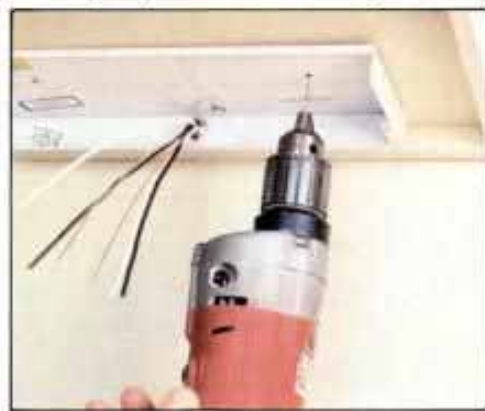
3 Strip off sheathing from cables and feed wires through connector. Locate fixture on cabinet, bore pilot holes and attach.
