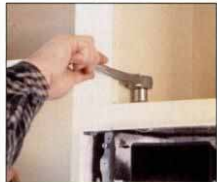
9 Attach microwave to cabinets above by sliding support bolts through prebored clearance holes and tightening securely.
