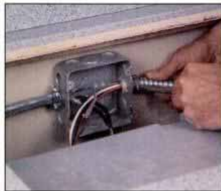
4 Slide oven part way into opening, then install cable connector and oven cable in box. Make connections with Wire-Nuts.
