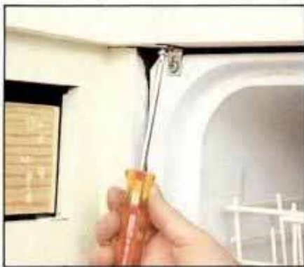
7 Remove screws that hold dishwasher to underside of countertop. Then pull unit—with drain hose—away from cabinet.
