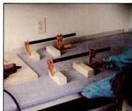
9 Temporarily attach clamping blocks to mating surfaces. Then apply fusion material and draw seam closed. Let dry for 2 hours.
