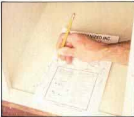
1 To install slide-out trash bag holder, position manufacturer's template on cabinet floor and mark screw hole locations.
