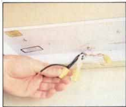
4 Cut and strip 6-in. pigtail wires, and join white wires together and black wires together using proper size Wire-Nuts.
