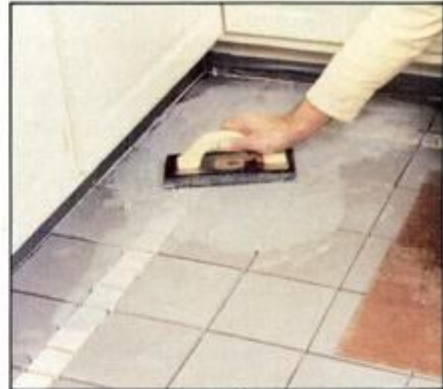
9 Once all tile is laid, let adhesive cure, then remove spacer blocks. Spread grout onto floor using rubber-faced trowel.
