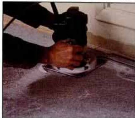
10 To make counter cutouts, use a router and straight bit with a ball-bearing pilot. Pilot follows cutout in substrate exactly.
