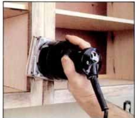
7 Thoroughly sand cabinets with 120-grit followed by 220-grit sandpaper for a smooth surface and good paint adhesion.
