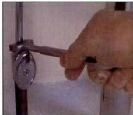
9 Cut faucet supply lines to proper length and slide ends into compression fittings on water supply shutoff valves. Tighten nuts.
