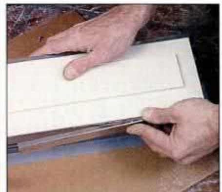
8 Install new panel so it's centered in opening and then attach trim strips by replacing screws. Reinstall access panel.
