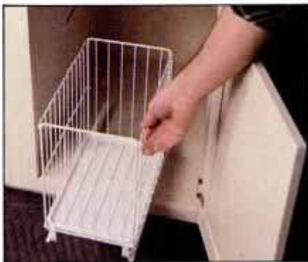
3 Assemble trash holder basket according to instructions and then slide assembly onto brackets. Place bag inside basket.
