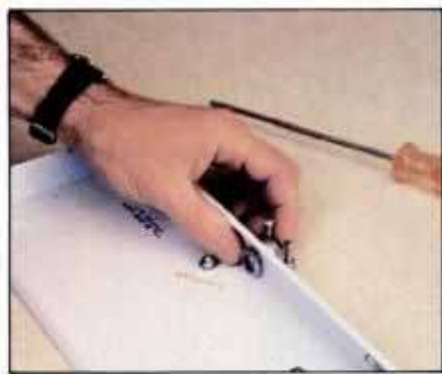
2 Determine most convenient location for entry of cables and remove knock-out plate. Install cable connector in hole.
