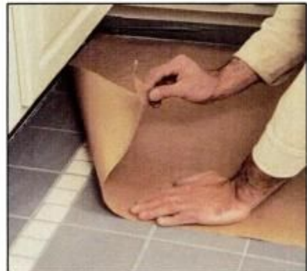
12 Because grout needs to cure slowly for best strength, cover floor with kraft paper to slow down drying process.
