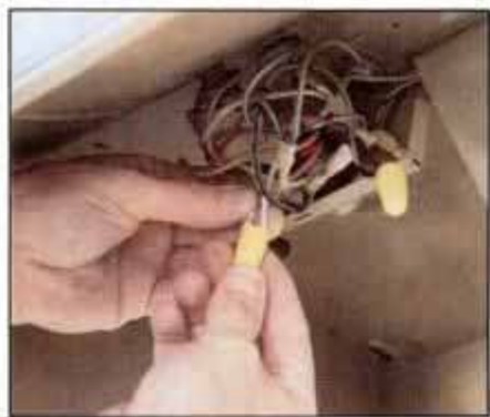
2 Disconnect all electrical connections and loosen cable connector. Support hood, then remove screws that hold it in place.
