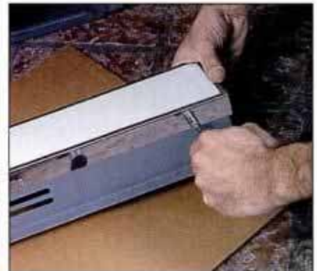
7 Remove trim strips from around access panel. Then remove decorative panel and any existing backing material behind it.
