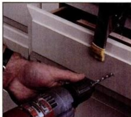
6 To install drawer pull, clamp alignment jig and backer block to drawer front and drawer box. Bore hole and install pull.
