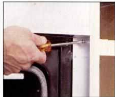
5 Slide oven completely into opening and check for level and plumb. Attach sides to cabinets with screws through oven flange.
