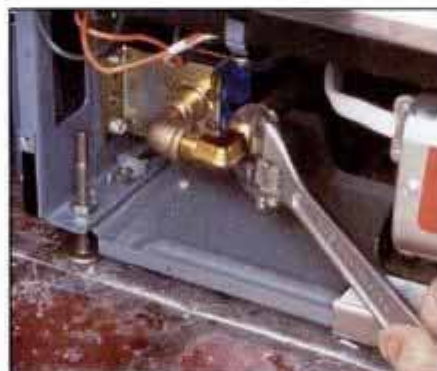
12 Connect water supply line to inlet valve with fittings recommended by manufacturer. Attach drain hose to disposer.
