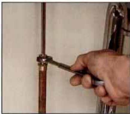
9 Shut off water at meter if necessary, and loosen compression fittings between water feed lines and sink supply lines.
