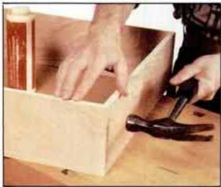
7 Construct new toe-kick assembly using \frac{1}{2} -in. or \frac{3}{4} -in. plywood. Miter corners, apply glue and join with finishing nails.
