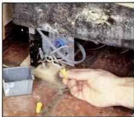
6 Shut off circuit power to unit and disconnect all electrical leads. Then shut off water supply and disconnect supply line.
