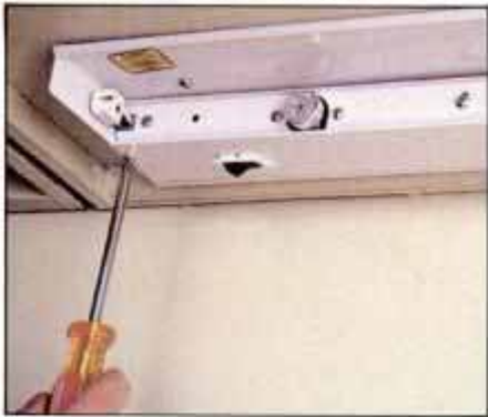
6 Carefully fold wires into wireway, then slide wireway into fixture. Align mounting holes and drive screws securely in place.
