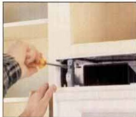
8 Hang microwave on mounting plate and temporarily support unit. Attach to plate by tightening screws at front of unit.
