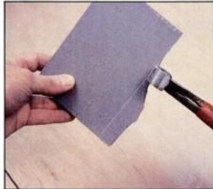
8 For irregular-shaped cuts—or straight cuts near edge—use tile nibblers. Remove small chunks until line is reached.
