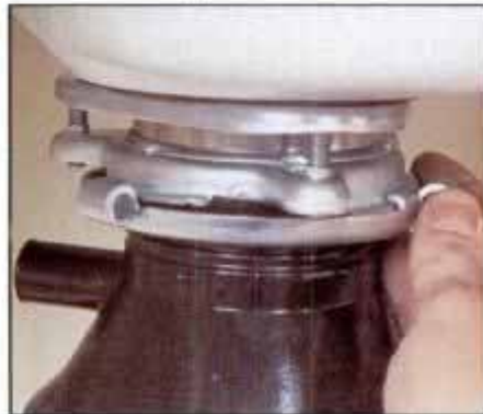
7 Lift disposer onto sink mounting ring, then rotate ring to clamp unit in place. Align drain connections before tightening.
