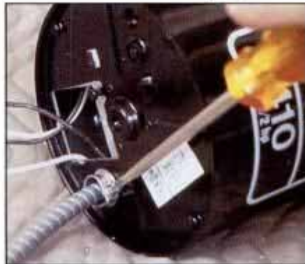
6 Remove disposer access panel and knockout plate. Install connector and power cable. Join wires with Wire-Nuts.
