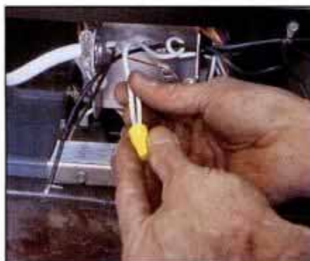
11 Connect ground wire to lug provided, then connect unit leads to feed wires. Whites together, blacks together.
