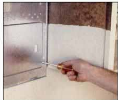
7 To install microwave, first attach mounting plate to wall. Drive mounting screws into wall studs for proper support.
