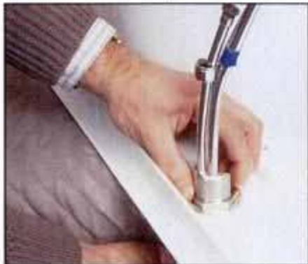
5 Install faucet by sliding through sink opening and tightening with retaining nut. Follow manufacturer's directions.
