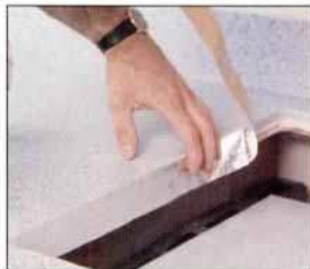
6 Check cooktop for fit in counter cutout, then remove and apply aluminum tape to counter edge to reflect heat. Install unit.
