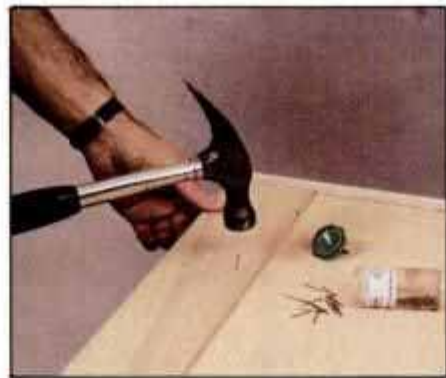
6 If back panel and face frame extend beyond sides, nail strips—cut to same thickness as space—to top and bottom of sides.
