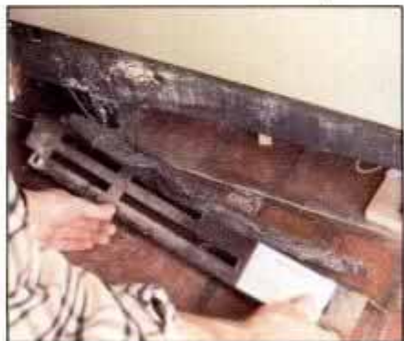
5 Remove access panel and lower trim panel (shown) to get to the electrical and plumbing connections underneath unit.
