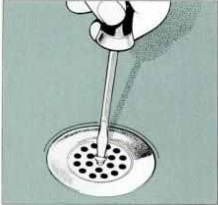
4 To remove hair, or plunge a tub with a plunger-type tripwaste, gain access to drain line by removing cover screen.
