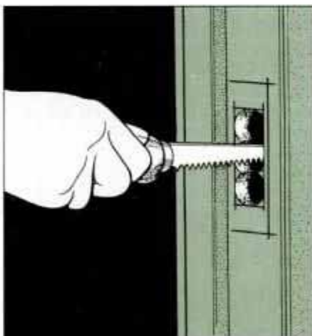
9 Using a drywall or keyhole saw, square the cut edges of the box recess. Test fit box to make sure it fits properly.
