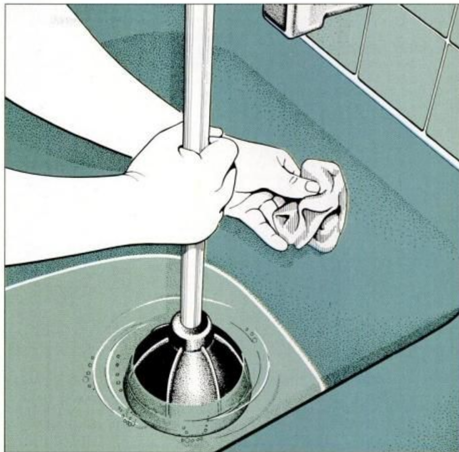
First step in clearing any clogged drain is to try plunging. For best results, be sure to plug any secondary passageways—like this tub overflow opening—with a damp rag.
