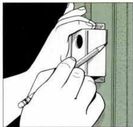
7 Place plunger-switch box against hinge side door jamb and door stop. Trace around perimeter of box using sharp pencil.
