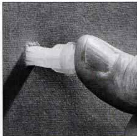
2 Insert folded anchor into hole and press until flush with surrounding surface.
