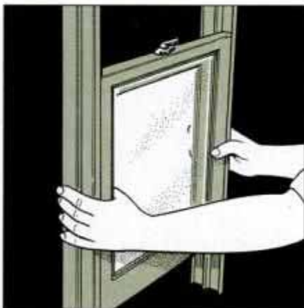
18 Aluminum replacement channels are available for standard-size windows. To install, channels are first fitted to both sashes.
