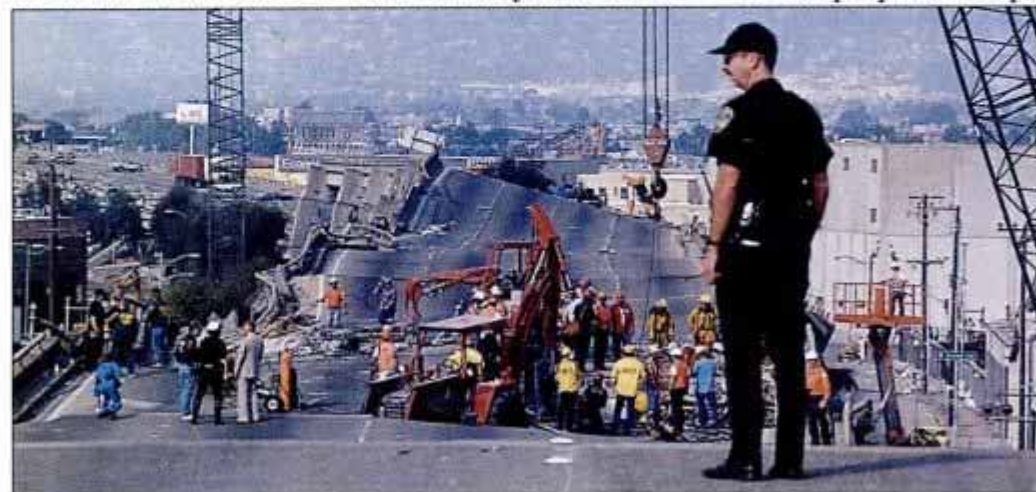
The deadly collapse of Interstate 880 in Oakland provides one example of a situation where early warning might have made all the difference in saving lives.
