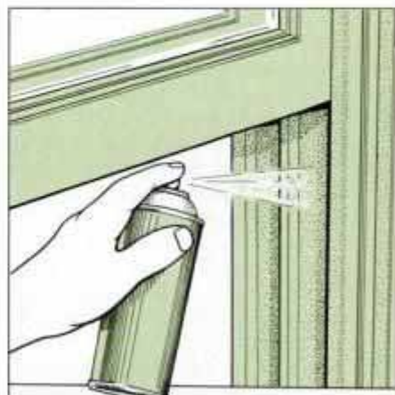
20 Use silicone spray lubricant to keep sash channels clean and smooth. It works on both wood and metal channels.
