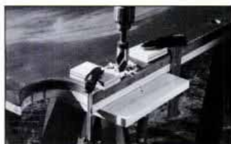
3 Bore rail bolt holes through the liner (slates come predrilled). Block ensures a clean hole where the bit exits liner.
