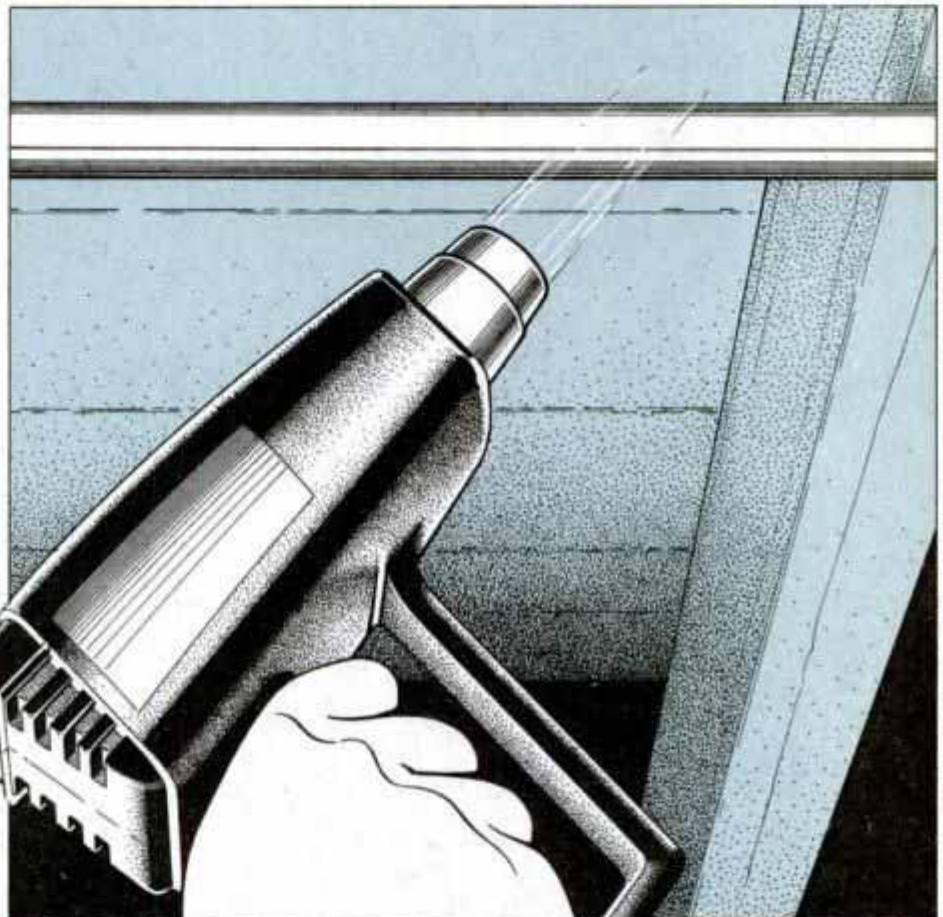
Sometimes the water inside a pipe will freeze and not break the pipe. If this happens, the fix is easy: Just heat the frozen section with a heat gun or soldering torch.
