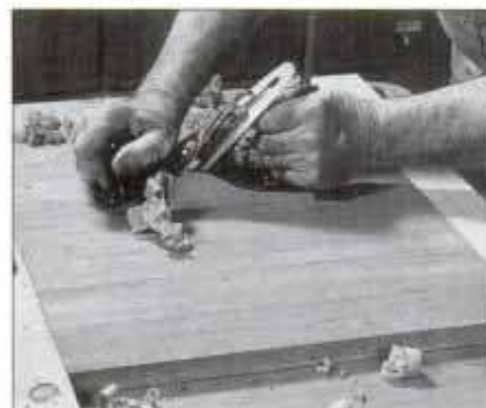
17 Use a smooth plane, with the grain, to finish. Keep the cutter sharp and set plane to produce the finest possible shavings.
