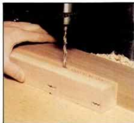
3 With scrap wood fence clamped to the drill press table, use ⅜-in. drill bit to bore overlapping mortise holes.
