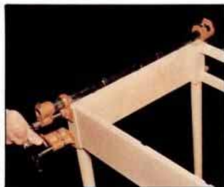
12 Complete leg-apron assembly by gluing and clamping side rails to legs. Measure opposite diagonals for square.
