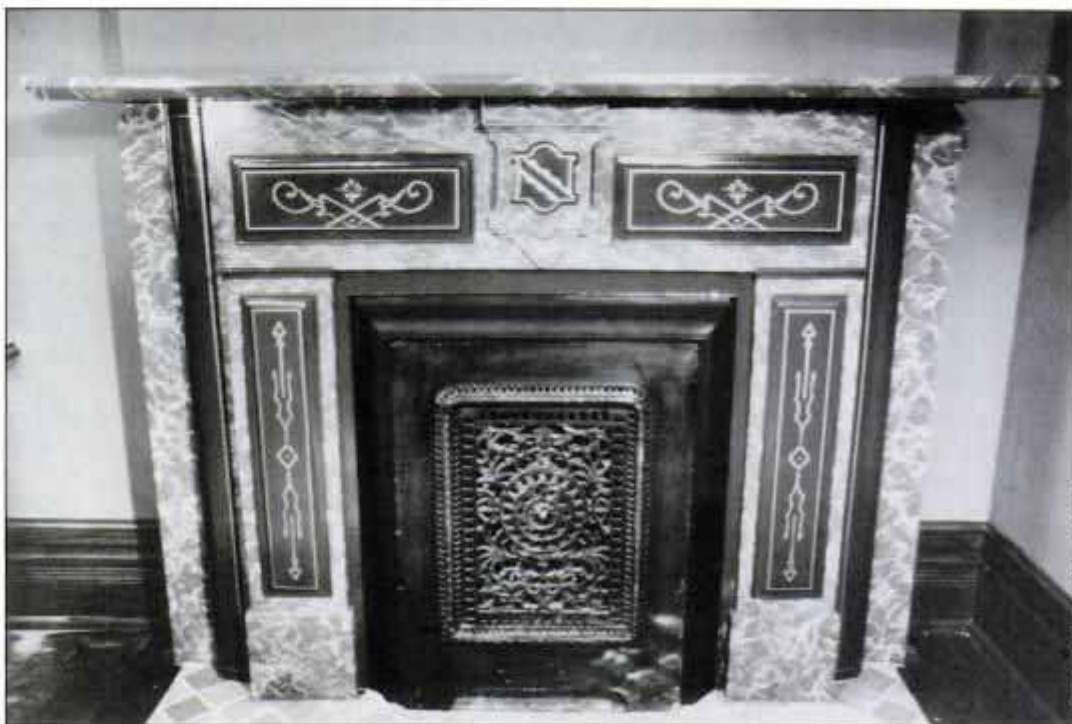
In the Victorian era, marbleizing fireplace mantels was especially popular. Often this faux finish was applied over cast iron or slate, with results that were astonishingly realistic.
