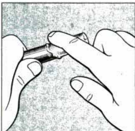
5 Apply noncorrosive flux to end of the cut tubing and end of the new sillcock.
