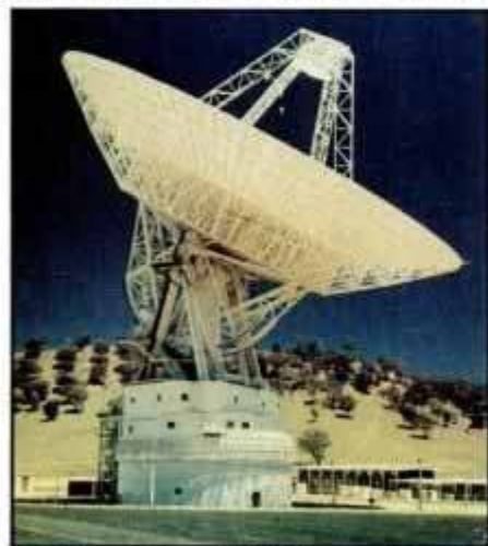
A vital component in the Voyager 2 mission is the Deep Space Network, a system of 70-meter receiving antennas like this one in Tidbinbilla, Australia.
