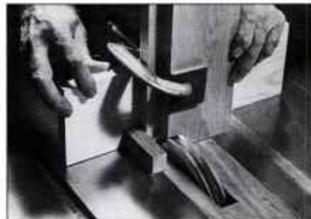
17 Clamp short apron to long apron and fence. Align edge of second piece with outer edge of first notch and make the cut.
