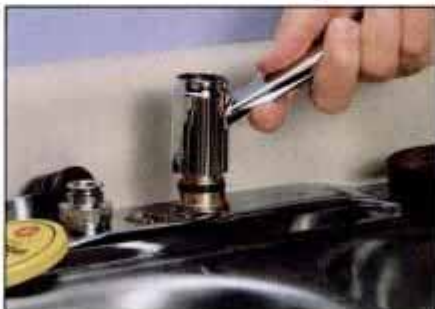
To remove a faucet spout collar, lift and twist until it comes free. It may require gentle prying with a flat blade screwdriver to loosen it.
