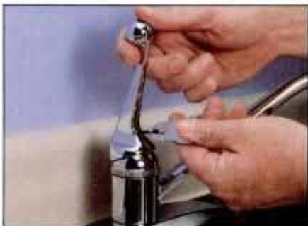
To remove the handle on a Delta single-lever faucet, tip the lever back and remove the Allen screw located on underside of arm.
