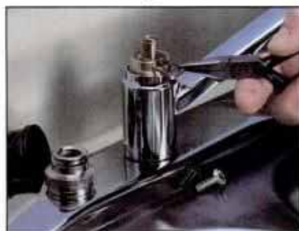
A brass retaining clip holds the cartridge secure inside the faucet body. Pull this clip out horizontally, using needle-nose pliers.
