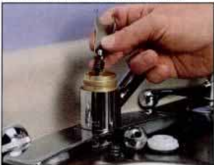
Remove the seats and springs using the Allen wrench that comes with each replacement kit. The new springs go into the ports first.
