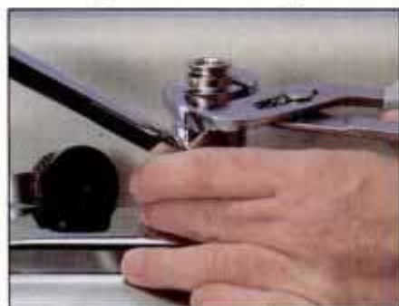
To free the fixture's cartridge, you must first loosen the pivot nut by turning it counter-clockwise with a pair of pliers.
