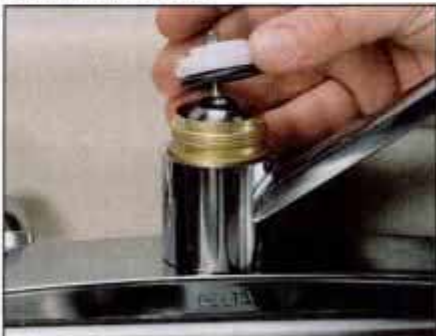
With the springs, seats and ball assembly in place, install a new cam assembly and replace the cap and lever handle.
