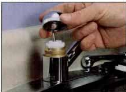
Loosen the threaded cap assembly with pliers and lift it off to reveal the cam and ball assemblies underneath.
