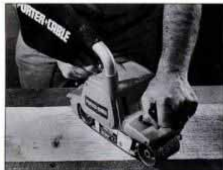
Although sanding across the grain isn't recommended ordinarily, it is a good way to remove stock quickly from rough lumber.
