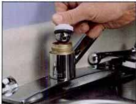
Lift the cam and ball assemblies out of the faucet body to reveal the seats and springs located underneath the ball.
