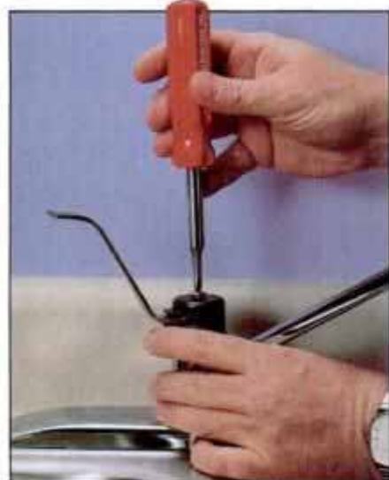
To remove a Moen faucet lever, loosen the screw on top of the handle and tip the lever back and up. Then pull off the lever.
