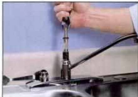
Once the clip is removed, pull the cartridge up and out of the faucet body. If the cartridge is stuck, wiggle it slightly.
