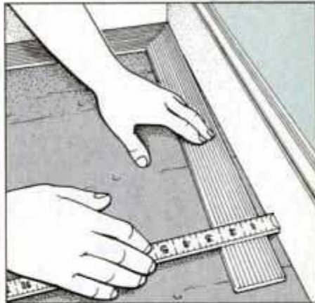
6 Use a framing square and ruler to determine how far out of square the corners are. Record the information on your drawing.
