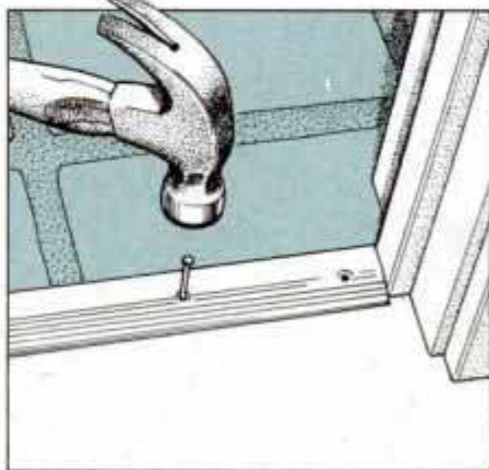
19 Where the new flooring joins another floor at doorways, nail a metal finish strip in place over the flooring edge.
