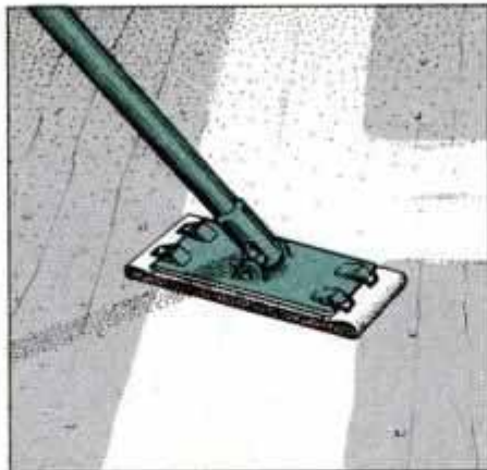
5 After the latex patching compound is dry, sand with 120-grit sandpaper. Using a pole sander makes it quick and easy.
