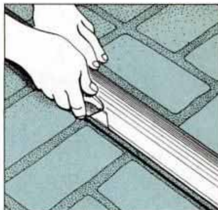
15 After installing both pieces with overlapping seam, use straightedge to cut seam along line in flooring pattern.
