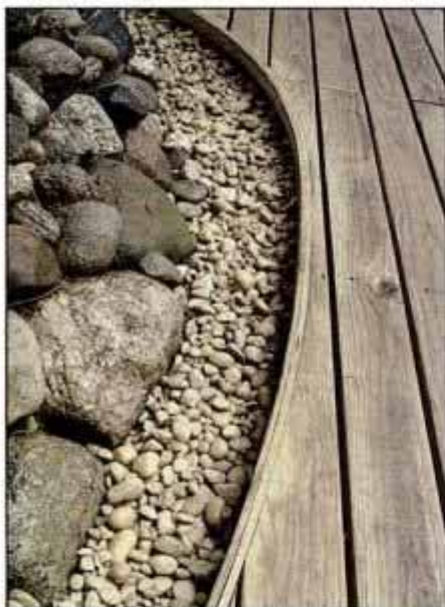
Edges of the walkway (above) are capped with edge banding to conceal the deck board ends and highlight the curve. Gravel next to walkway makes lawn maintenance easier. The overall shape of the walkway is determined by yard and landscaping features such as a rock garden (below).
