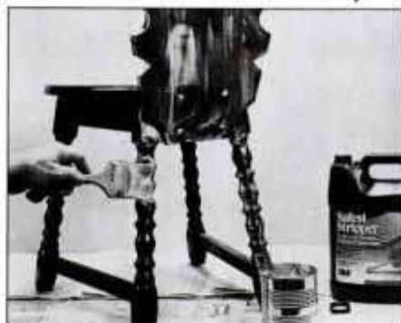
Apply stripper to work with paint brush. A 2- to 3-in.-wide brush works best. Spread newspaper under piece to protect floor.
