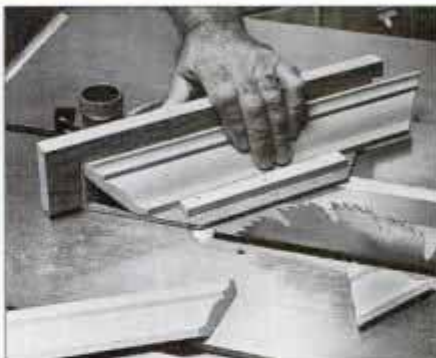
Build this simple jig to cut compound angles on crown molding. Wood-strip stop block props up molding, holds it at proper angle.
