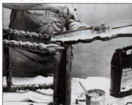
Stripper softens paint without blistering. It can be left on for long periods without drying out. Remove paint with a putty knife.
