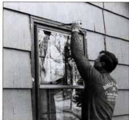
2 Remove nails that hold window in place from outside. Be careful not to split brick molding. Then pry out window unit.
