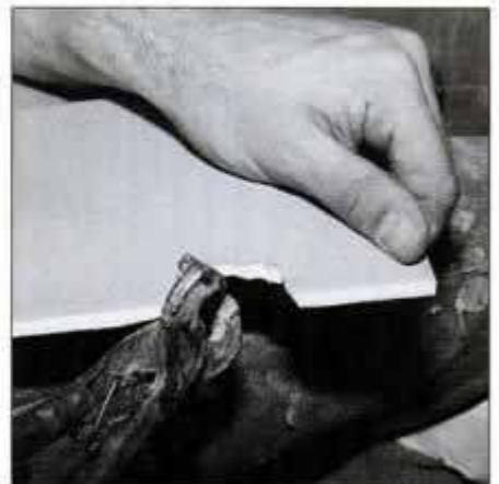
6 Make irregular cutouts with tile nippers. Simply snip off small pieces of tile until you get desired shape. Do not take big bites.
