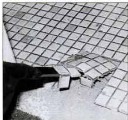
3 Use a flat bar to lift off floor tile or vinyl flooring. Be sure to wear eye protection to prevent injury from the tile chips.
