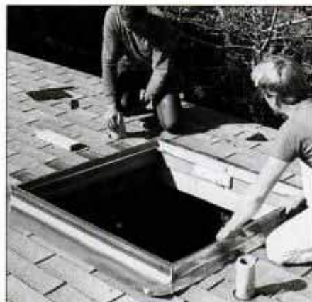
5 Slide skylight frame into place, then flash according to manufacturer's directions. When done, install the window panel.
