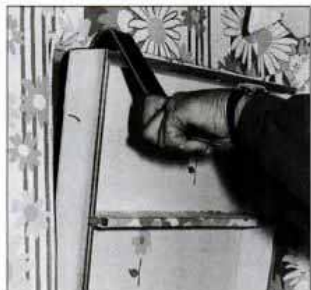
2 Carefully remove any mirrors in the room, then pry out the medicine cabinet. Be sure to remove screws that hold cabinet first.
