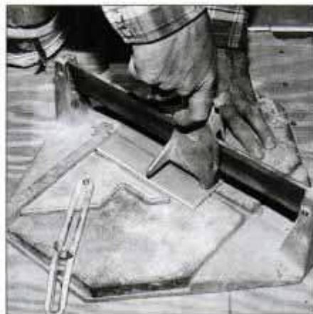
5 Make straight tile cuts with tile cutter, an inexpensive rental item. Cutter scores tile with sharp wheel then snaps tile in two.
