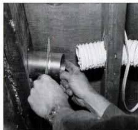
4 Slide support plate over hood pipe and push tight against joist. Then slide hose over pipe and attach with duct tape.
