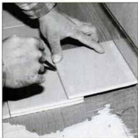
4 To measure perimeter tiles, lay tile to be cut over last full course. Push next tile against wall and scribe top tile for perfect fit.
