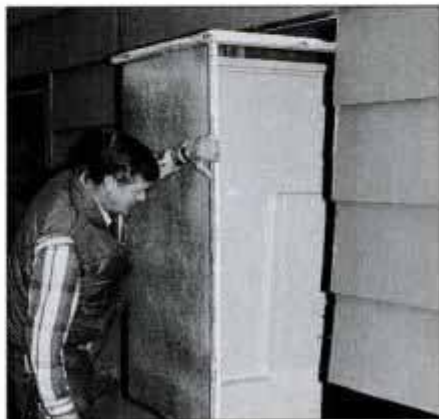
5 Slide the new tub enclosure through the opening, being careful not to scratch the fiberglass. Reinstall the framing and siding.
