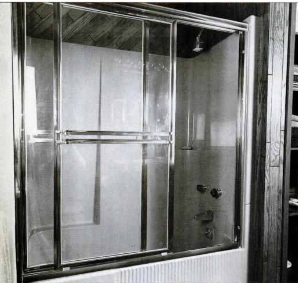
Oversized tub and shower enclosures, like this fiberglass unit, are roomy and luxurious. But they're too big to move through your house. Here's the way to make them work.
