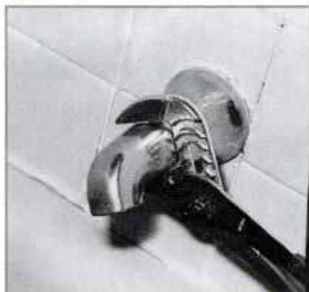
1 First remove all faucets, escutcheons and other fittings, like a tub spout, that are accessible from the outside of the fixture.
