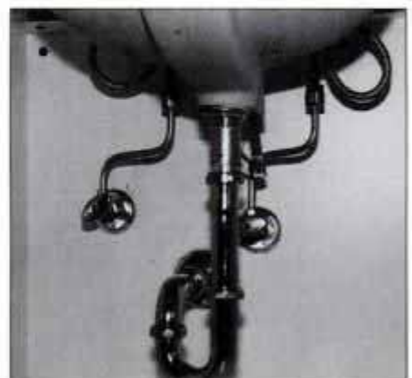
5 Use trap and tailpiece to attach sink drain to waste pipe. Then connect supply lines to shutoff valves on hot- and cold-water pipes.
