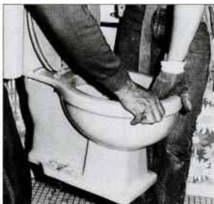
There's nothing written in stone about the location of any plumbing fixture. They are all movable, with varying amounts of difficulty. Here's what's involved in moving a toilet.
