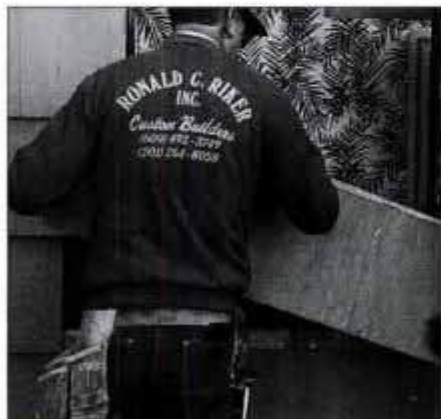
3 Carefully remove the siding from below the window, starting at the window opening and working down to the bottom plate.
