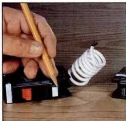
GFCI breakers are identified by a test button and a dedicated neutral conductor, which on this model is the coiled white wire.
