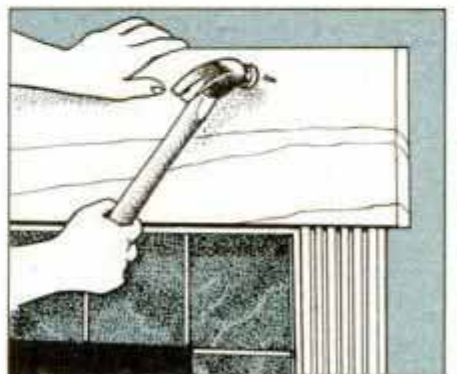
9 After cutting the 5/4x10 entablature stock to exact length, sand ends and secure it to the wall with 10d finishing nails.
