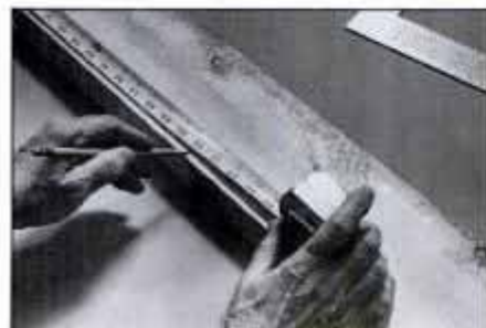
7 To mark rafter length, measure top edge of board starting at plumb line, not cut line. Mark edge at proper length.
