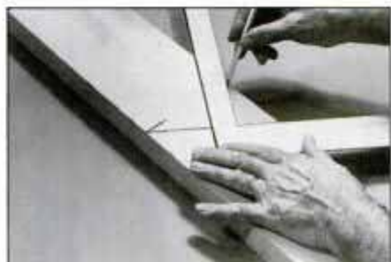
9 To mark bird's mouth, hold square perpendicular to plumb line and where length of cutout equals width of wall plate.
