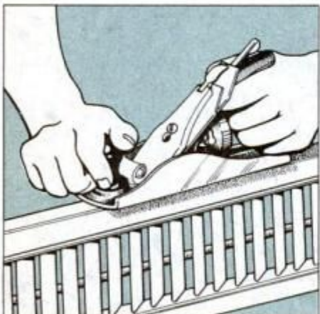
5 A sharp hand plane removes stock when trimming. Remove an equal amount from all shutters for uniform appearance.
