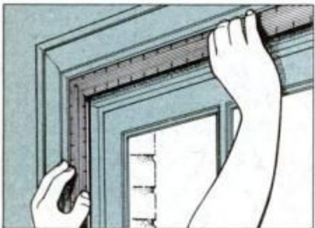
3 Check the window jambs for square. Severely out-of-square jambs make an outside, casing installation a better idea.
