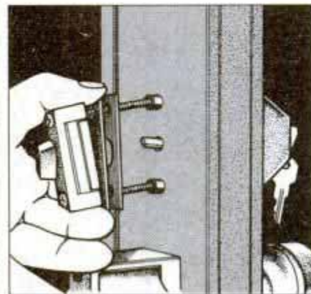
11 Install the dead bolt opposite the key lock. Be sure that the flat spindle is seated properly in the center of the bolt assembly.
