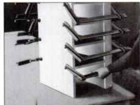
5 Quickly clamp assembly together before glue starts to dry. Be sure to check for square and readjust clamps if necessary.
