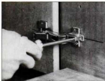
10 Hang cabinet doors by sliding hinge into mounting plate on case side. Tighten hinge screws, then close door and check fit.
