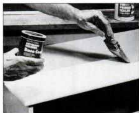
10 Begin the graining by applying a colored base coat over the primer. Base coat is a quick-drying satin latex paint.
