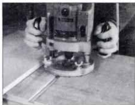
1 Cut side panels to size, then lay out and rout shelf dadoes in sides using \frac{3}{4} -in. straight bit and straightedge guide.
