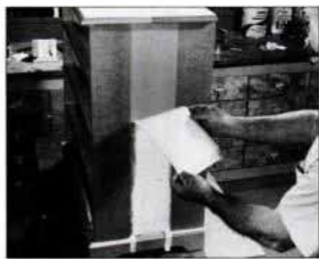
16 After each section is dry, remove adjacent masking and mask off finished areas. This creates the look of individual boards.
