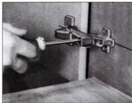
11 To obtain proper fit, turn adjusting screws as required. Screws can move door in and out, up and down, and side to side.
