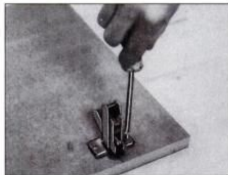
9 Carefully locate hinge positions on back of doors, then bore hinge-mounting hole. Push hinge into hole and attach with screws.
