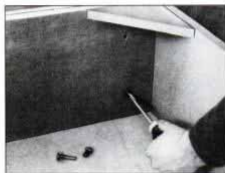
16 Temporarily install connecting screws to secure both bases. Check for flush alignment along top edges, then remove screws.
