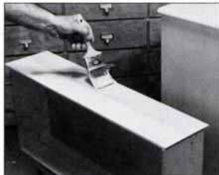
2 Stenciling requires a smooth, flat background. Latex satin-finish enamel is applied over the primer. Avoid glossy paints.
