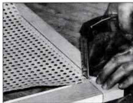
5 Secure cane by first stapling two corners. Place staples along rabbet 1 in. apart and avoid distorting cane pattern.
