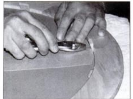
15 When installing wedges, protect the mirror back with a piece of thin cardboard. Press \frac{5}{8} -in. wire brads in place with pliers.
