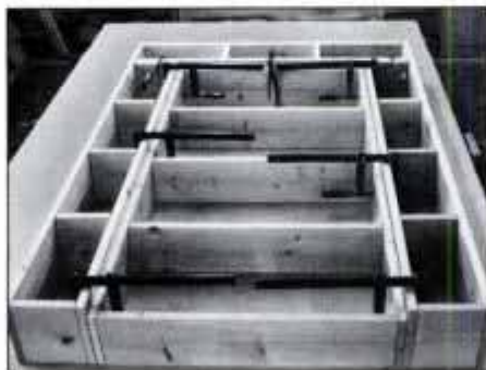
2 Temporarily secure the four base frame subassemblies with clamps. Then, join the frames together with 2-in. No. 8 fh screws.
