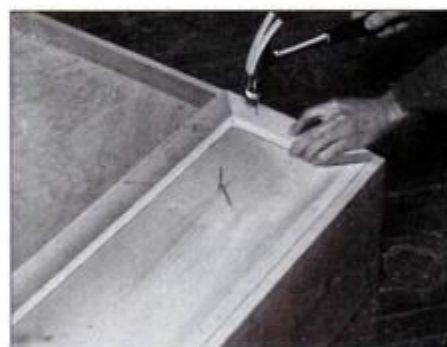
9 Cut all spacers and shelves to size and secure first row to base with 3d finishing nails. Spacers are set back \frac{3}{4} in. from edge.
