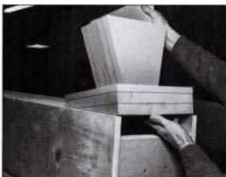
17 After the top band assembly has been secured to the top spacers, secure keystone supports in recesses at band frame ends.
