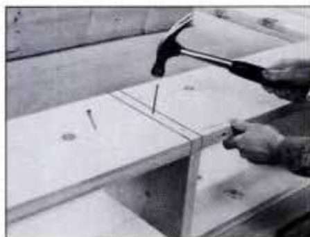
1 Lay out assembly lines on base frame sides. Fasten sides to cross blocking with 8d common nails. Use three nails per joint.
