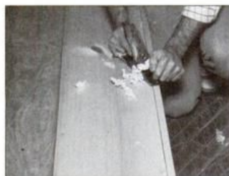
4 If the upper edges of the side trim are not flush with the faces of the caps, carefully trim the edges with a sharp hand plane.
