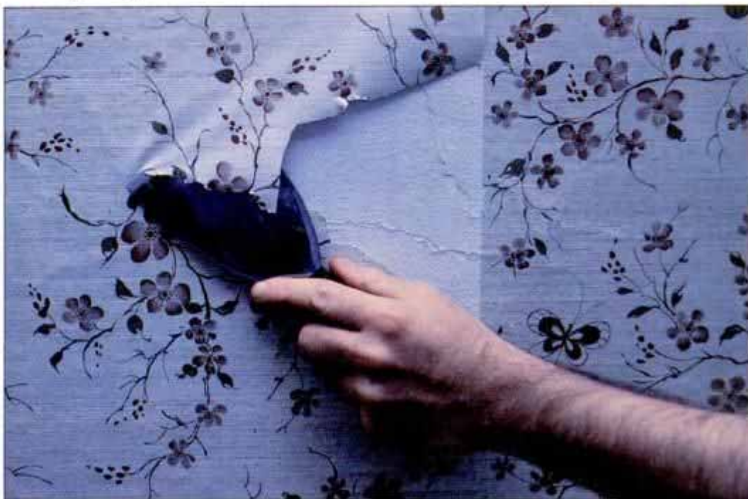
Removing old wallpaper is crucial to the success of a new papering job.
