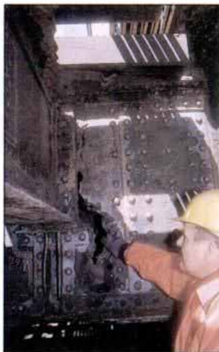
Connecticut's Mianus River bridge (above) collapsed after corrosion consumed a support pin. New York's aging Williamsburg Bridge (above right) suffers from a litany of abuses ranging from rock-salt runoff to piled-up pigeon droppings. The result: holes in support girders (right) that forced temporary closing.
