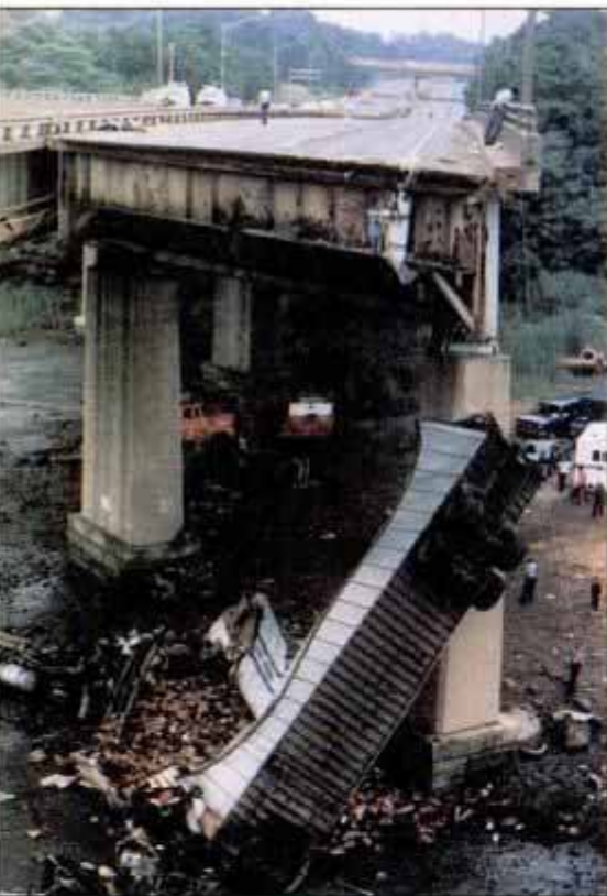
Connecticut's Mianus River bridge (above) collapsed after corrosion consumed a support pin. New York's aging Williamsburg Bridge (above right) suffers from a litany of abuses ranging from rock-salt runoff to piled-up pigeon droppings. The result: holes in support girders (right) that forced temporary closing.
