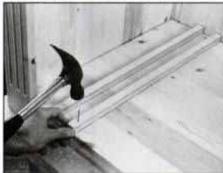
11 Use 3d finishing nails to attach strips to the cart bottom. These act as spacers for holding trays and the case partition.
