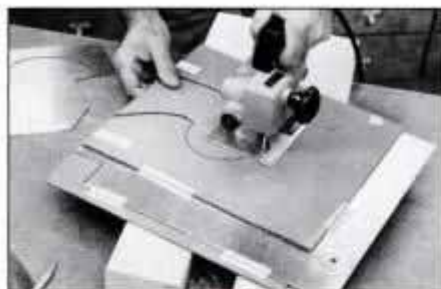
To obtain clean, chatter-free cuts in sheet metal, place it between pieces of cardboard or 1/4-in. plywood. Support work on 2x4s.
