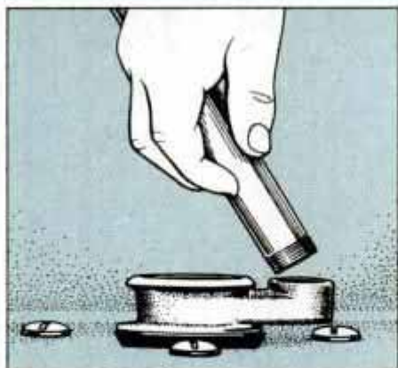
13 If you find a broken overflow tube, pull old tube out, pry threads from the flush valve, and thread a new tube in place.
