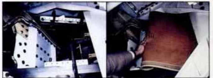
At left, wing hinge-pin laid open to show fuel lines and electrical conduits. At right, Kevlar blanket covering vulnerable components.
