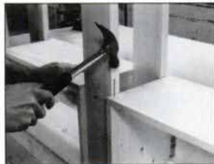
8 The second row of shelves rests on shelf supports. Make sure shelf edges are flush with the supports. Glue and nail in place.
