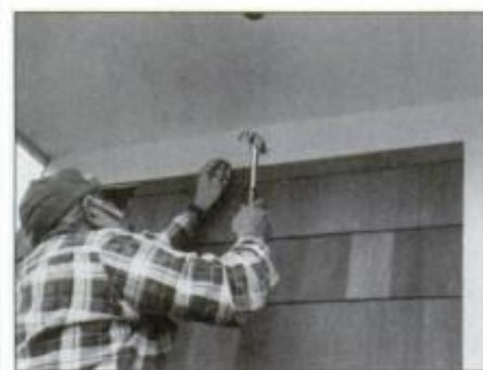
15 Install top course. Position nails near bottom edge, and along top edge. Nail through siding and wood backer strip.
