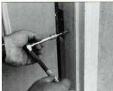
10 Adjustable Jamb-Jacks secure the door. Use a ratchet wrench and special driver (provided) to screw bolt into stud.
