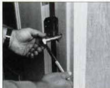
11 Reverse the special driver in the wrench and use it to adjust jambs in or out until the door and frame align perfectly.
