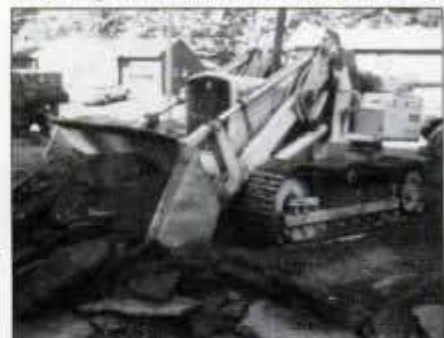
1 Track-driven shovel dozer tears out old driveway. Dozer's front bucket scoops asphalt chunks and drops them in truck.
