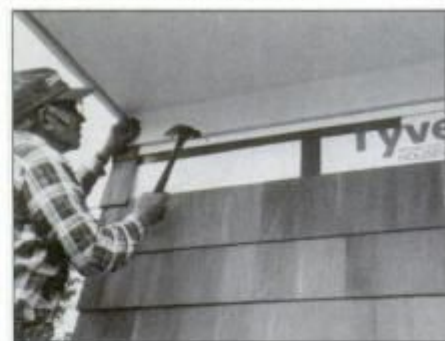
14 Before installing the top course of the siding, nail a 1/2-in.-thick x 1 1/4-in.-wide wood strip to house under the frieze board.
