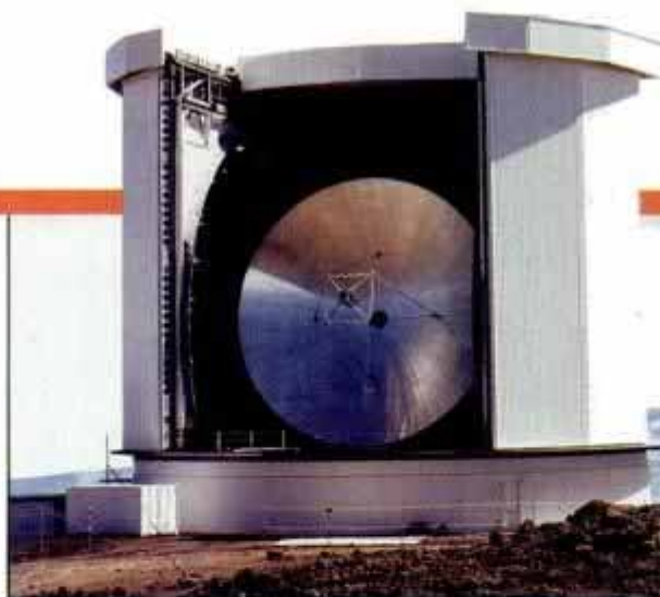
Telescope's housing gives clear view while blocking winds.
