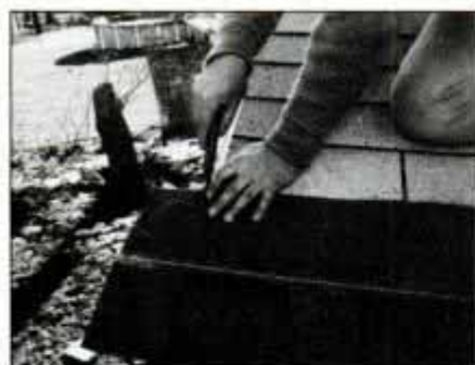
4 Mark cut line on first shingle of second course using sharp utility knife. Cut line should be flush with aluminum edging.
