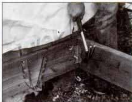
2 Nail the first and last joists to end of ledger and then install a metal corner bracket (as shown) to strengthen the joint.
