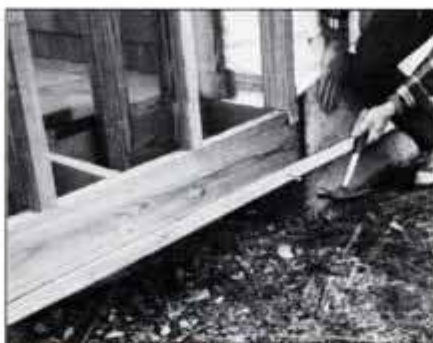
16 Before installing siding, nail a 1/2-in.-thick starter strip along the bottom of header joist. Continue the strip onto house.
