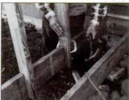
9 Prebore the 2x4 studs and then nail them to the joist 16 in. on-center. Note that the stud is notched to fit onto the 2x8 joist.
