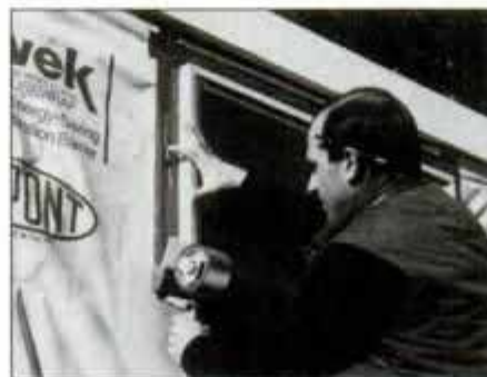
3 For a totally energy-efficient seal, apply 3M's sheathing tape around windows and doors. Use tape to seal all Tyvek seams, too.
