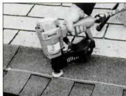
7 Air-driven nailer is a rental item that saves a lot of time and energy. To use, just press nose against shingle and pull trigger.
