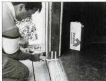
7 Apply two parallel beads of butyl caulk along the sill and up the sides about 3 in. This will stop air and water infiltration.
