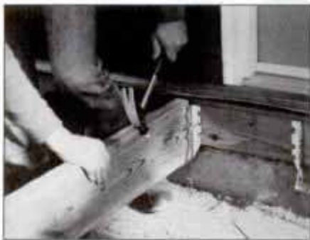
6 Drop the joist into the hanger and nail the hanger to ledger first. Then, nail hanger to the joist with the nails provided.
