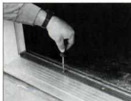
13 Door features an adjustable sill that stops drafts. Loosen screws slightly to raise sill. Then, close door and check the seal.
