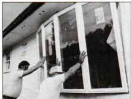
5 After rough opening is framed out, install the window. Two people are needed to hold unit while it's secured from inside.
