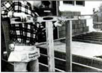
10 Clamp opposite stud in place and level across tops. Inside studs aren't notched, but instead, nailed flat against the 2x8 joist.
