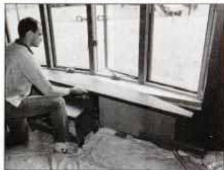
8 Unit has factory-fitted seat board. Apply stain or paint before installation. If needed, rip seat board flush with interior wall.
