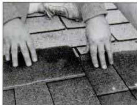
3 Begin second shingle course by abutting full shingle to first alignment slot that appears in top edge of shingle below.
