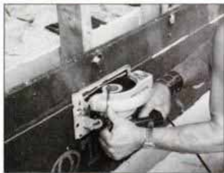
2 Make a plunge cut—3 in. below rough opening dimension—into each stud. Use reciprocating saw to cut stud completely.
