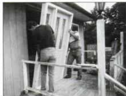
8 Position unit in the opening, sill first, and then tilt in the top. Note that door and sidelight come assembled as one unit.
