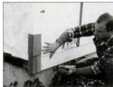
9 Start first course with a prefabricated corner. Be sure corner is plumb on both sides and hangs just below the starter strip.
