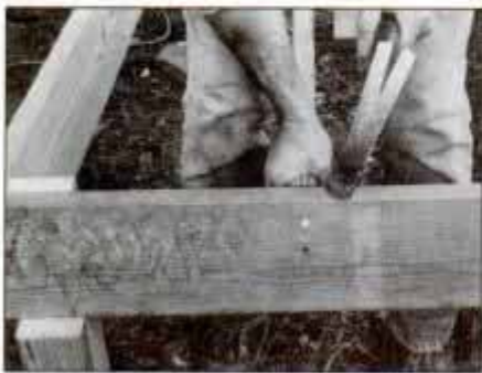
7 Fasten other end of joist by simply nailing through the galvanized header and into joist end. Use three 16d nails per joist.
