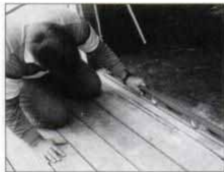
6 Check sill for level. It must be level for door to operate properly. Also, check to be sure sides of opening are plumb.
