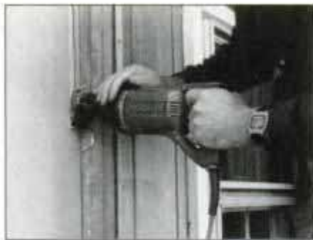
4 Cut away the interior wall with a reciprocating saw. Hang a drop cloth on inside wall and execute cut from the outside.
