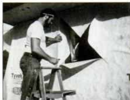
2 Then, slit the Tyvek at each window opening from corner to corner. Fold Tyvek into the opening and reinstall the window.
