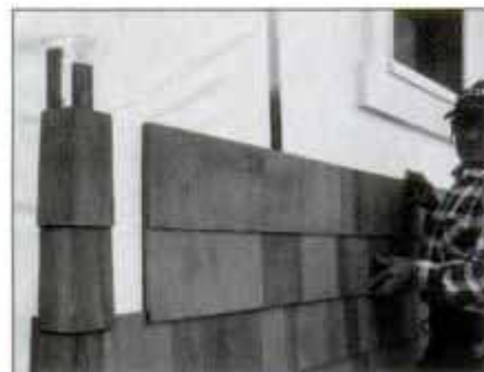
10 Continue by installing a corner followed by a course of siding. Note: Shims are often necessary to keep the corner plumb.
