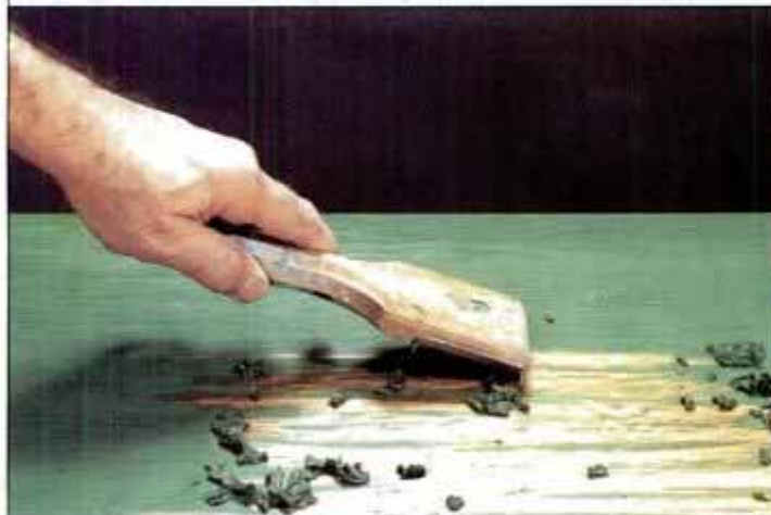
A hand scraper removes paint well but can scratch and gouge wood.
