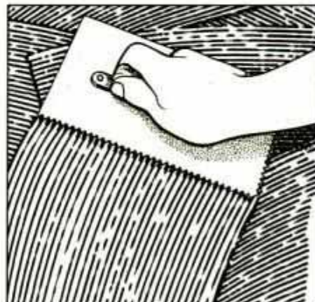
12 Apply mastic in small sections using notched trowel held at 45° angle. Use a sweeping motion to get best coverage.
