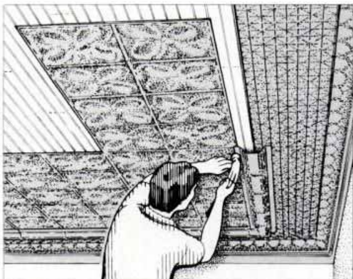
Components can be attached directly to wood ceilings or to furring nailed over a plaster or drywall. The arrangement shown consists of 2x8 panels surrounded by a cornice and crown molding.
