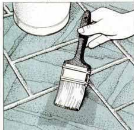
17 If you want to seal the floor, wait 30 days then brush on a thin coat of commercial sealer. Let dry and apply second coat.
