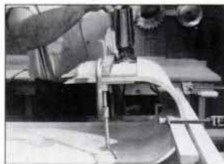
13 Clamp the slats together with a straightedge to guide the sabre saw. Before unclamping, mark the rear cut-off line.
