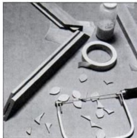
13 Cut 1/8-in.-thick plywood splines shaped to fit the slots. Use a yellow glue and tape the joints until the glue sets.
