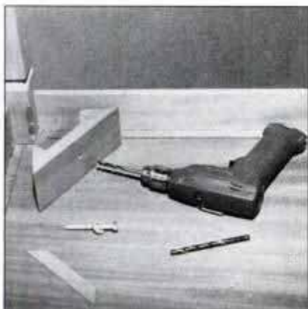
11 Corner blocks add rigidity to the frame. Secure to the legs with \frac{5}{16} \times 3\frac{1}{2} -in. lagscrews and to the apron with glue.
