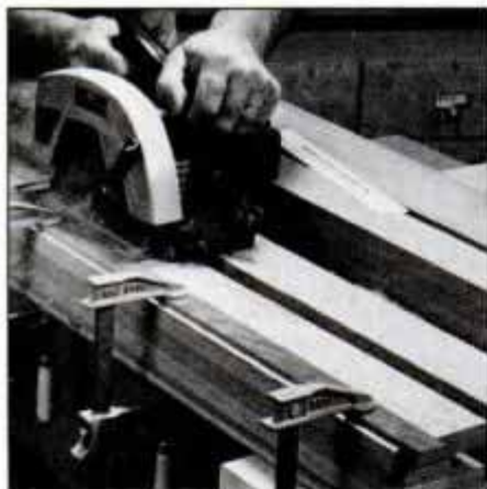
1 Glue up the leg stock and use a circular saw guided by a straightedge to rip. Scrap panel underneath protects the bench.
