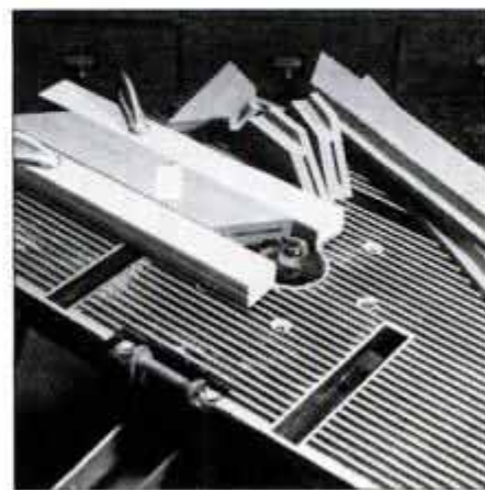
12 Cut joint slots with slotting bit. Guides keep the slot from going through corners. Tape short sections for safer operation.
