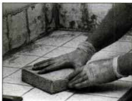
Wipe off excess grout right away using sponge and fresh water. Buff off the dried haze after several hours with coarse cloth.
