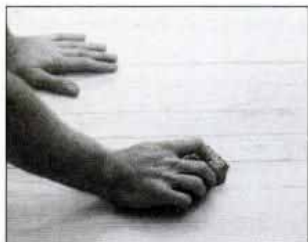
Sand floor lightly to remove any raised grain from "pickling" process. Vacuum carefully, then wipe thoroughly with a tackcloth.
