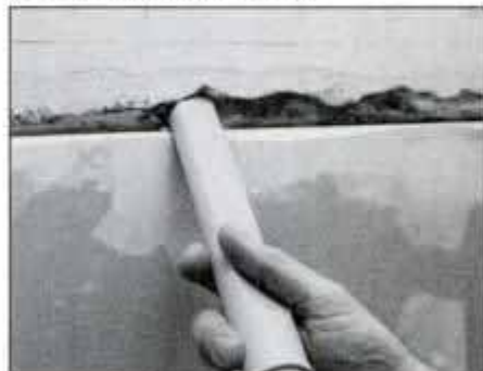
Make large patches using drywall that matches the thickness of old plaster. Clean joints with vacuum cleaner before finishing.
