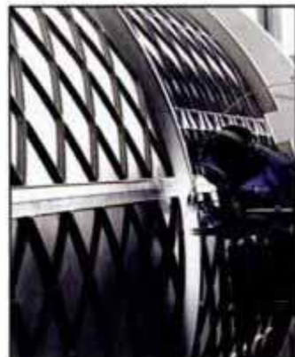
Welding the Space Station.
