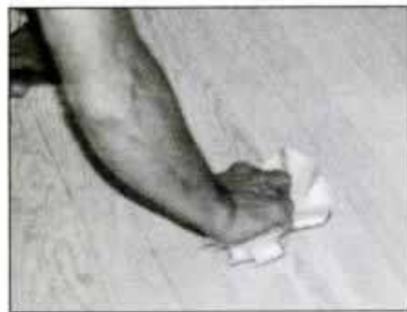
Use a latex woodgrain filler that matches wood floor to fill cracks and joints. Wipe off any excess with a damp cloth.
