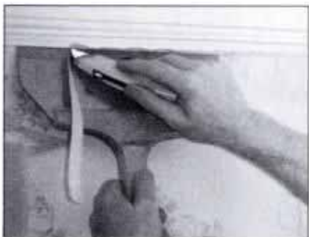
Use metal straightedge, like a 10-in. taping knife, to press paper against trim or ceiling. Then cut edge with sharp utility knife.
