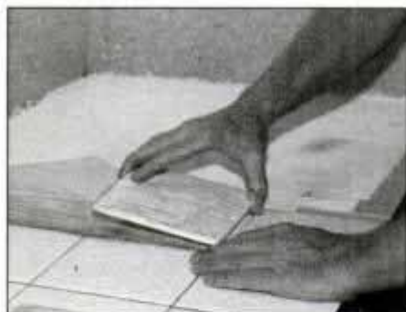
Set tile into mastic with a slight twisting motion to imbed the underside tile grooves in mastic. Do not slide tile in place.
