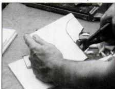
Use nibbling pliers to shape curves around sink cutout. For best results, work slowly, removing just 1/4- to 1/2-in. at a time.
