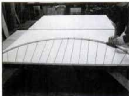
13 Transfer the spindle positions to a layout board. Clamp the bow in place and mark the spindle-hole positions on bow.
