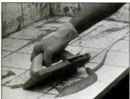
After mastic has set for 24 hours, apply grout using rubber float. Work grout well into joints, holding float at 45° angle.
