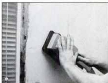
Sand surface smooth using fine-grit sandpaper. Sears vacuum sander attachment (shown) eliminates nearly all the dust.
