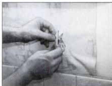
Cut small "X" in wallpaper above receptacles and other fixtures. Then carefully smooth the wallpaper and trim away any excess.
