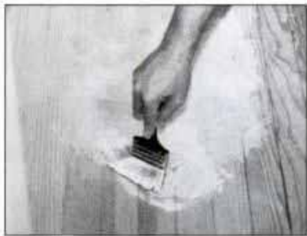
Apply flat white latex paint to floor, scrubbing in with an inexpensive brush. Work in floor sections that are about 2 ft. sq.
