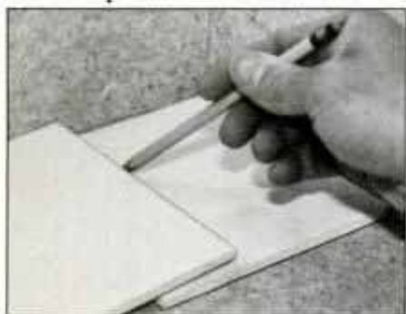
Position the last tile—which must be cut—against counter end, under previous tile. Trace cutting line onto tile with a pencil.
