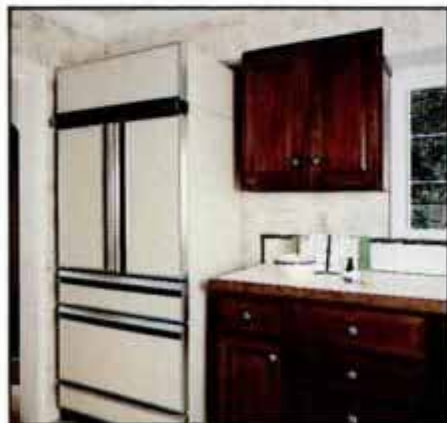
New, shallow-profile refrigerator fits behind doorway casing, creating custom look.
