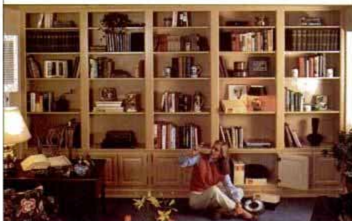
Bookcase wall: Popular project needs molding for tight ceiling fit.
