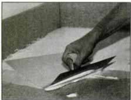
Spread premixed ceramic tile mastic onto countertop using a notched trowel held at a 45° angle. Make sure to spread it evenly.
