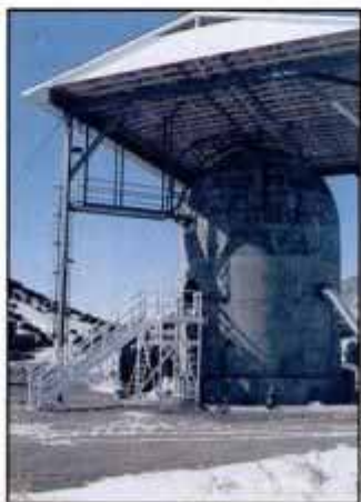
The reactor model will be pressurized to 115 percent of designed capacity.
