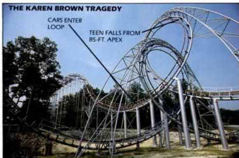
The twin Lightnin' Loops roller coasters at Great Adventure in New Jersey stand empty following the death of 19-year-old Karen Brown. Her safety bar somehow closed behind her and her body was pitched from the top of the highest loop. Could an overreliance on computer safety checks have led to operator complacency? Opposite: A roller coaster's vast potential for fun is revealed aboard the Tidal Wave at Great America in Chicago.
