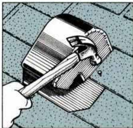
7 Fasten vent cap with roofing nails fitted with rubber washers. Nail through flashing and apply roof cement to nailheads.
