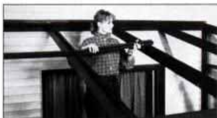
After attaching the rafters to the wallplate and the front rail, install the purlins. Simply push down to lock the purlins in place.
