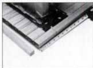
After sawing off the oak trim, cut the door to length. Reattach the trim with glue and nails.
