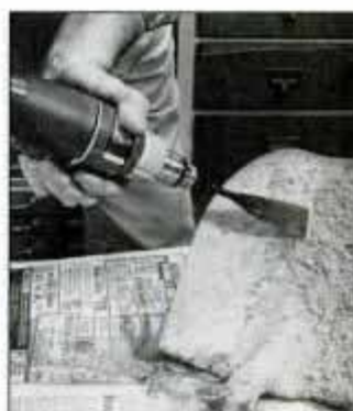
The \frac{1}{4} -in.-wide rigid scraper works fine on rough work like chipping off hardened concrete.
